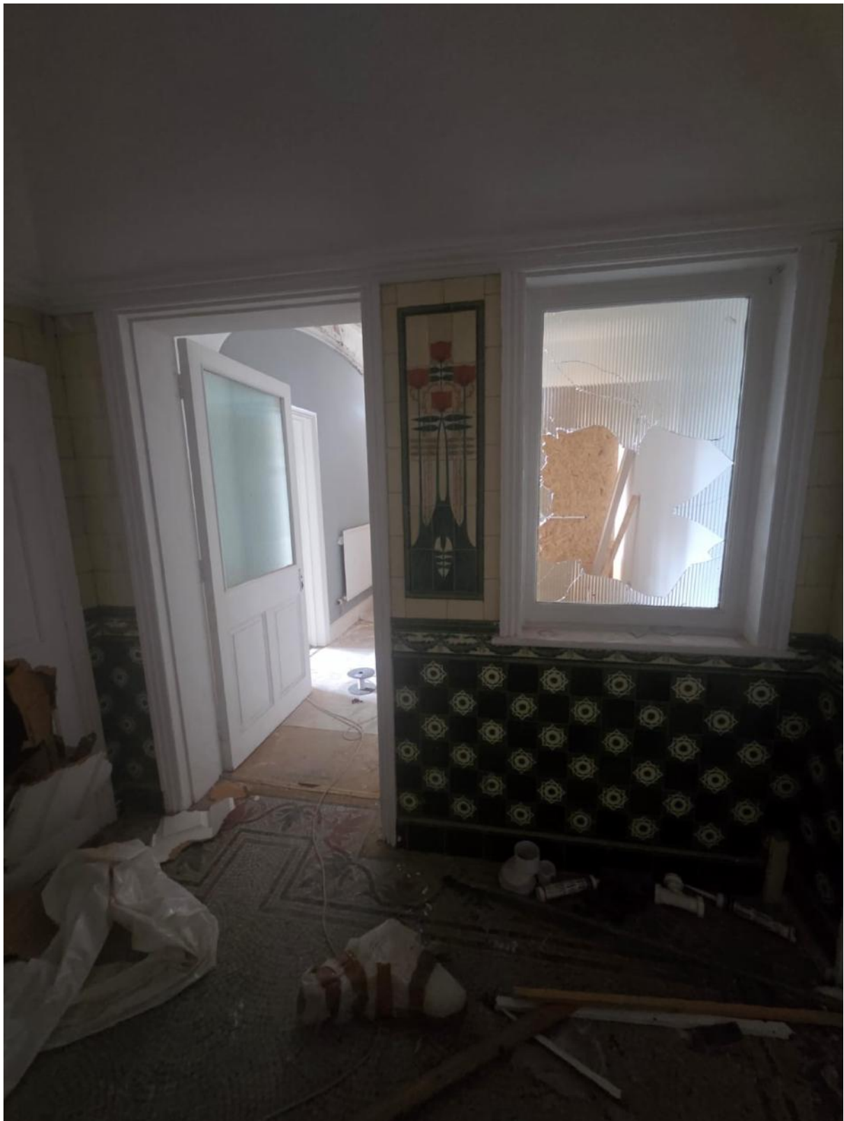
Leading to Shower Room Area
