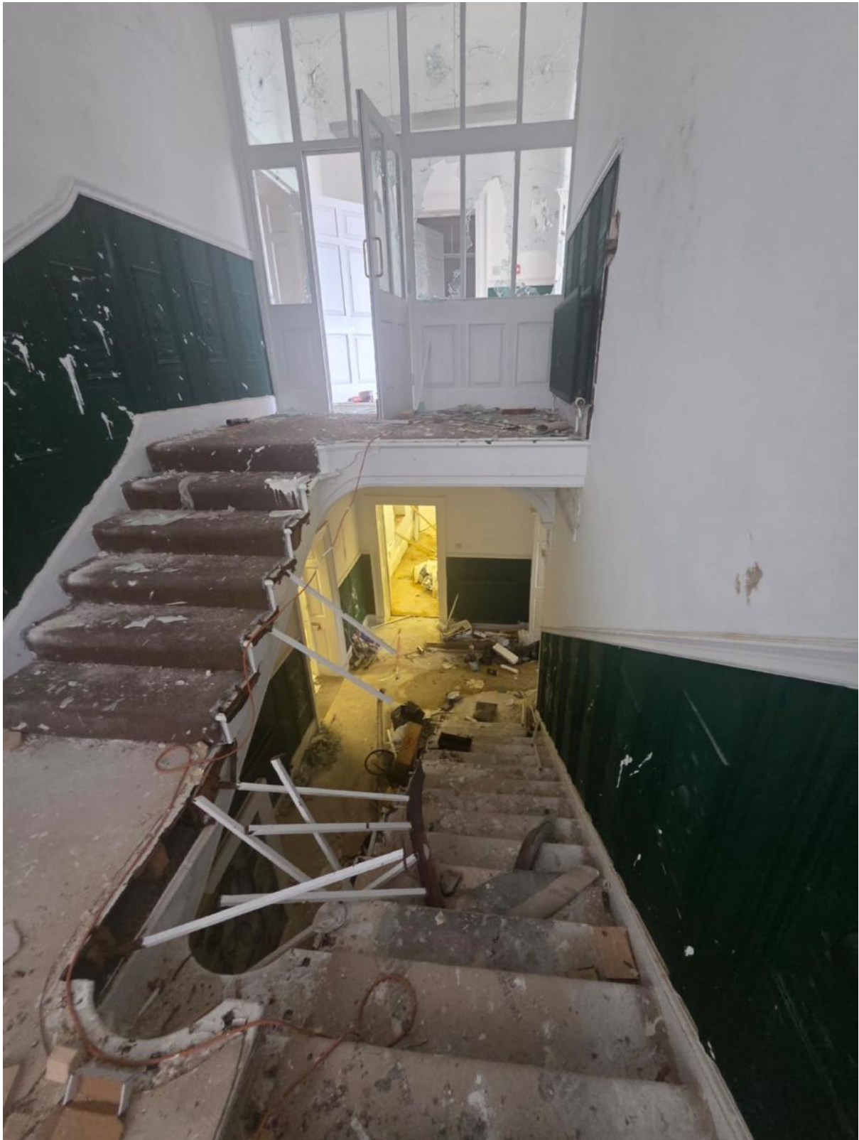
Ground & First Floor - Staircase Landing
