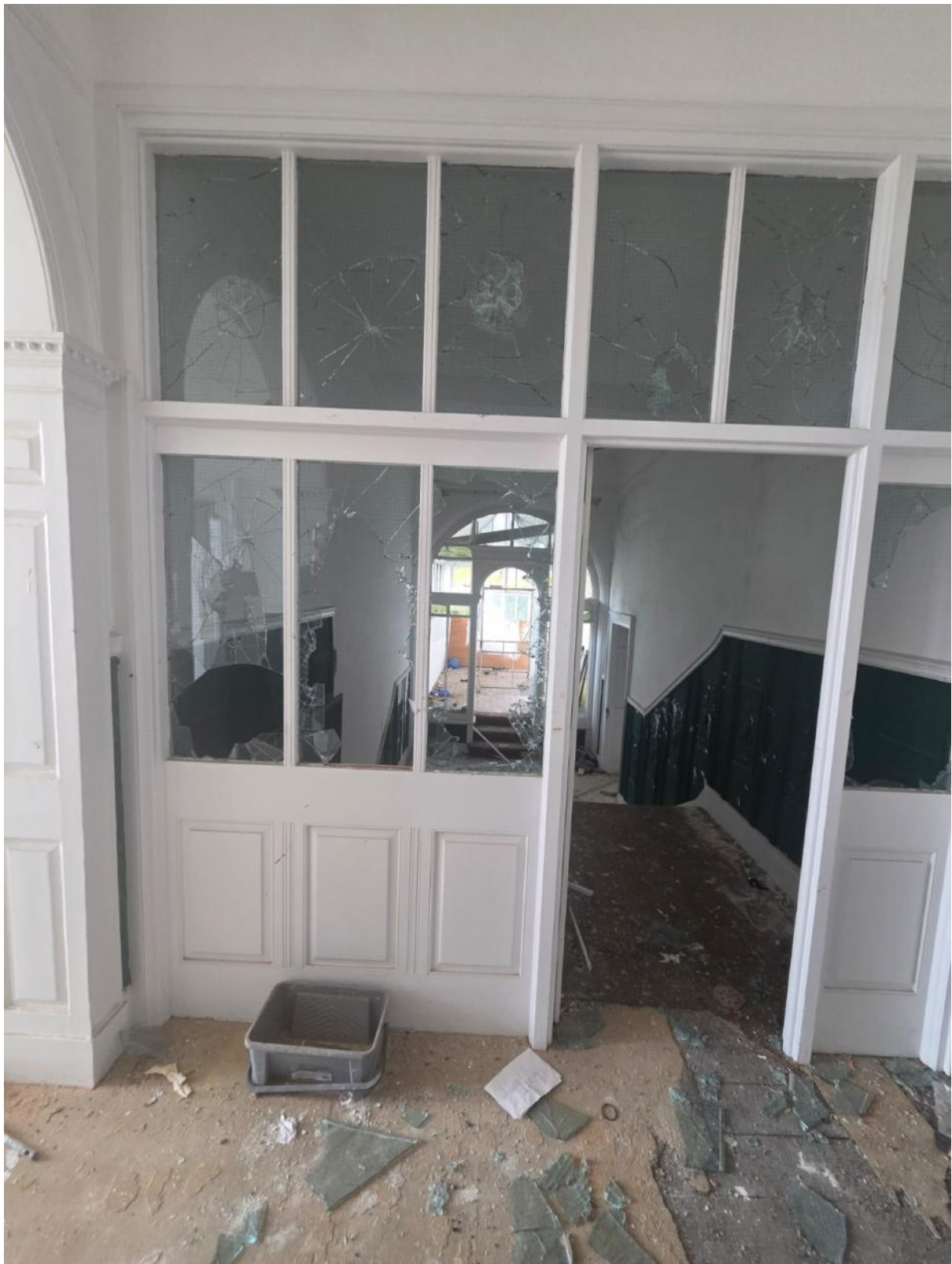
Landing to Corridor
