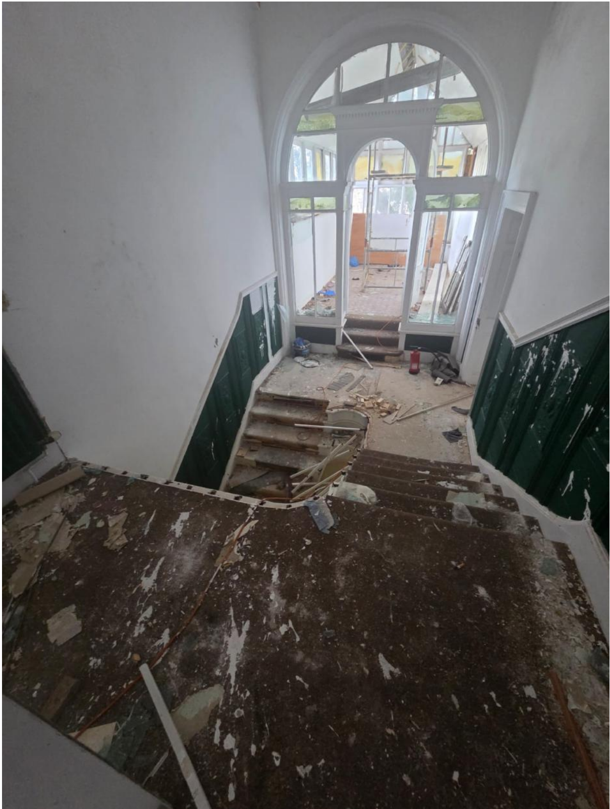
Staircase or Landing Leading To Staff Office
