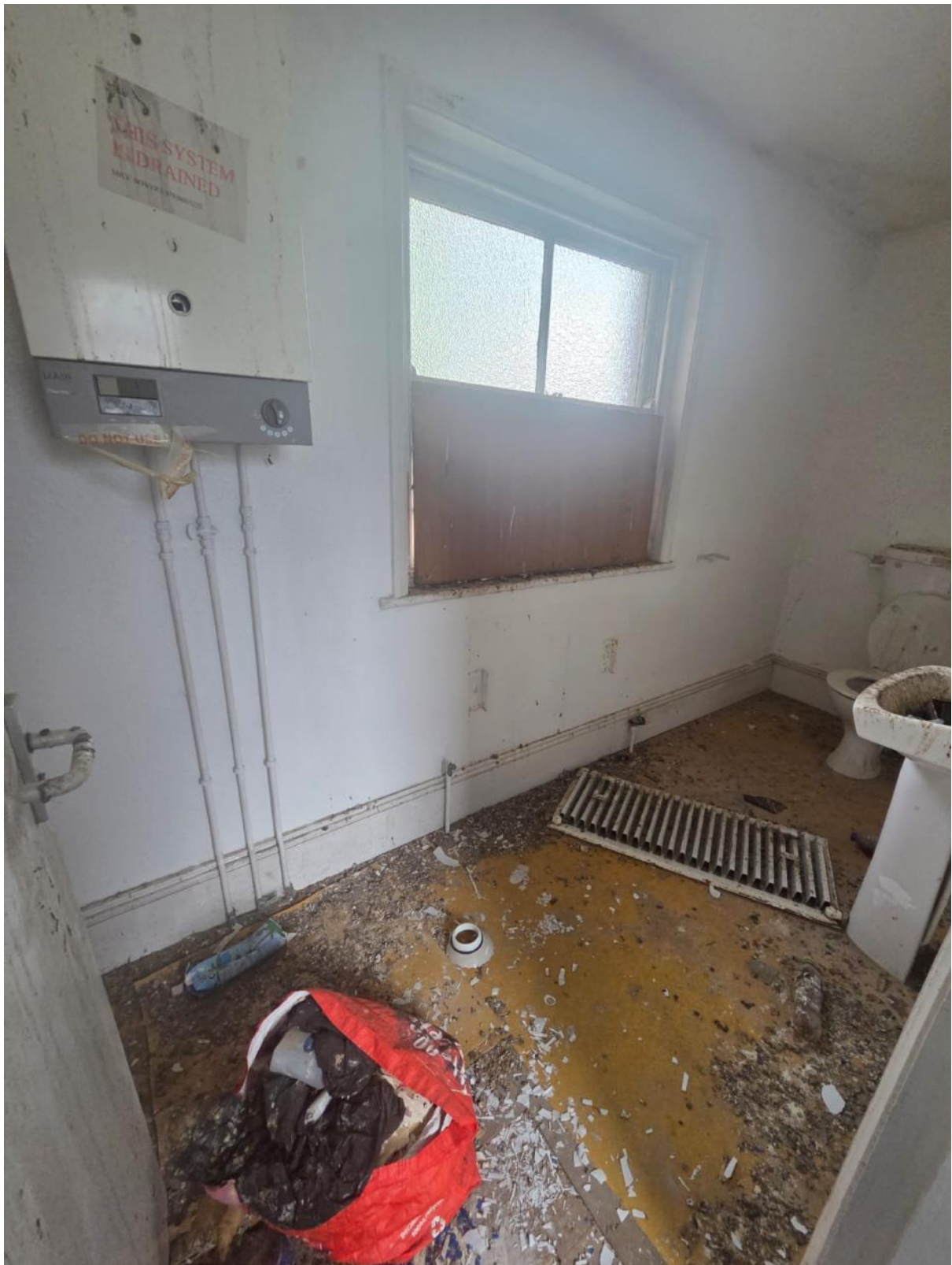
Up & Down New Stair Case Leading To Ground Floor
