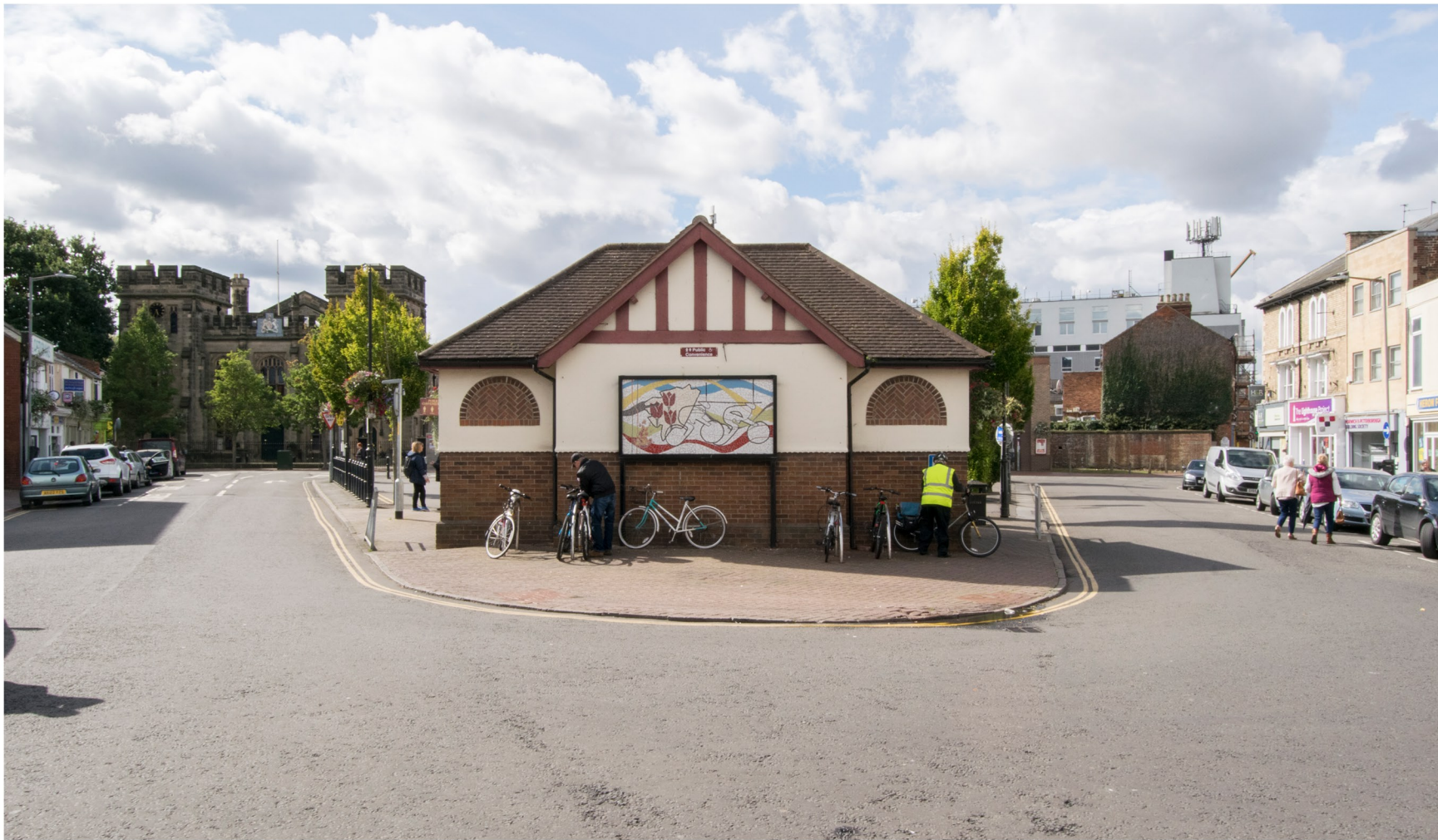
Existing view looking west towards site
