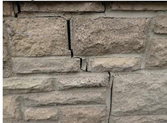
The natural stone is pitch-faced and semi-coursed. The existing stone is to be carefully taken down, cleaned and used in the reconstruction.
