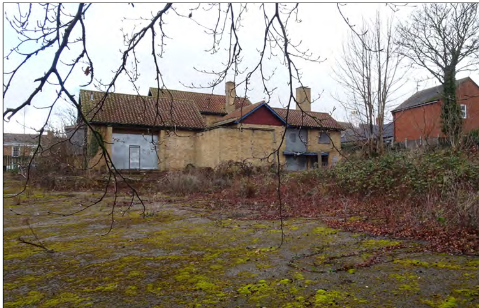
A: The site looking northwest
