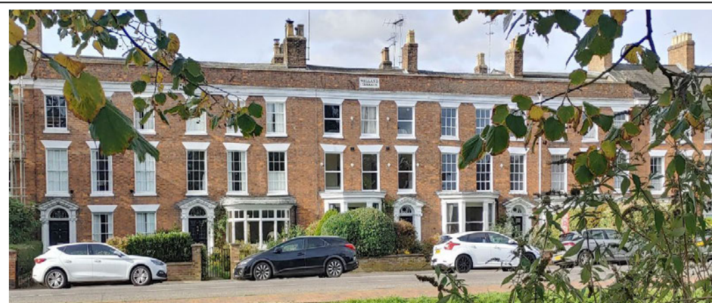
Welland Terrace – Central Section
