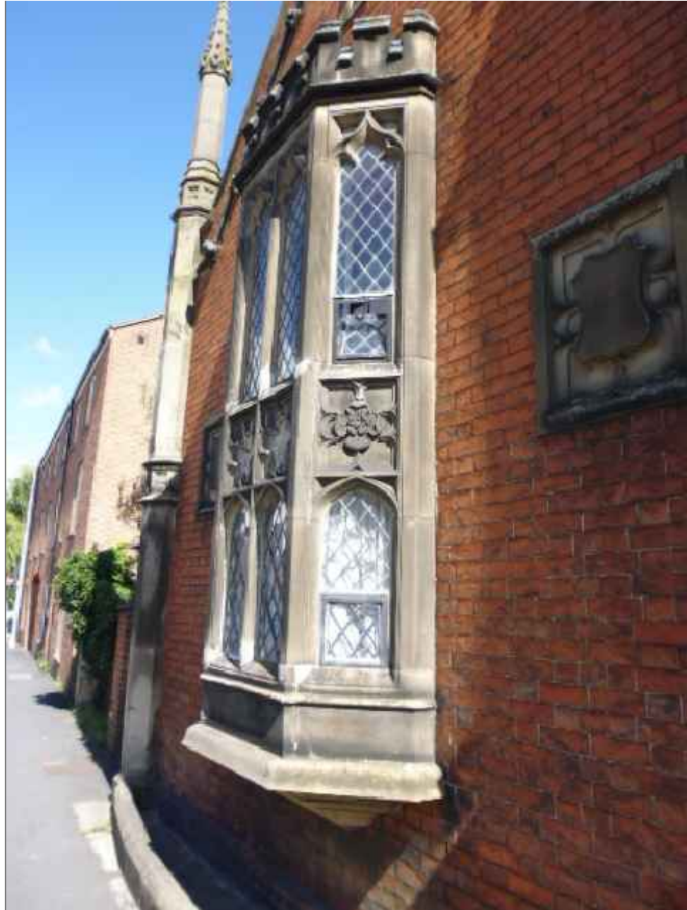
Photo 1 - Projecting Stone Bay - Properties 1 & 2.
