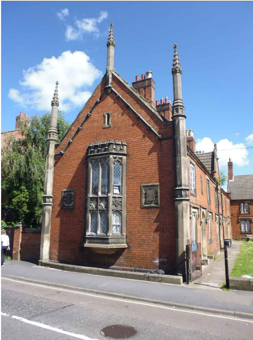
Photo 4 - West Block Gable- Properties 1 to 6
