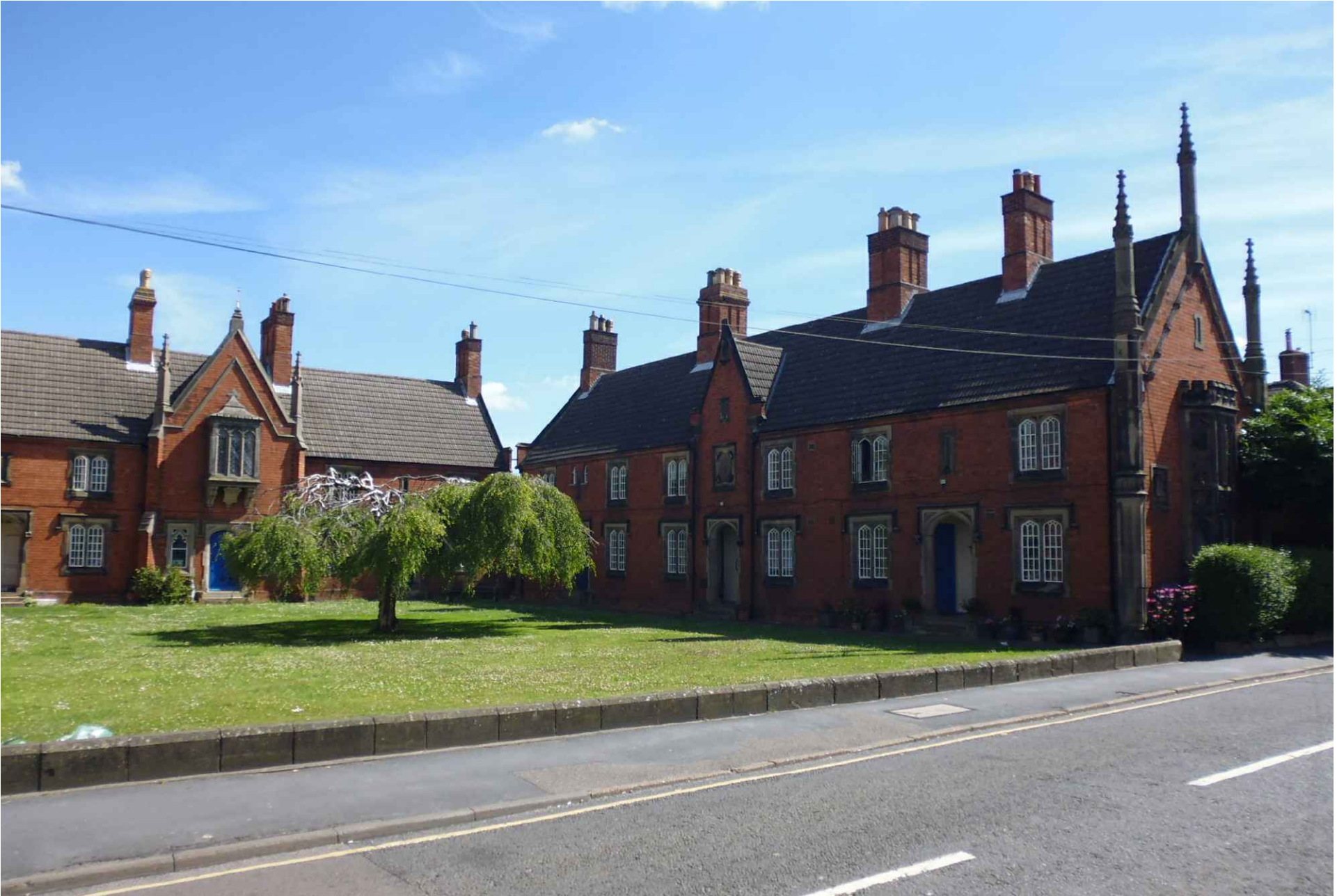
Photo 2 - Part North Block and East Block - Properties 9, 10, 11 and 12 to 16.
