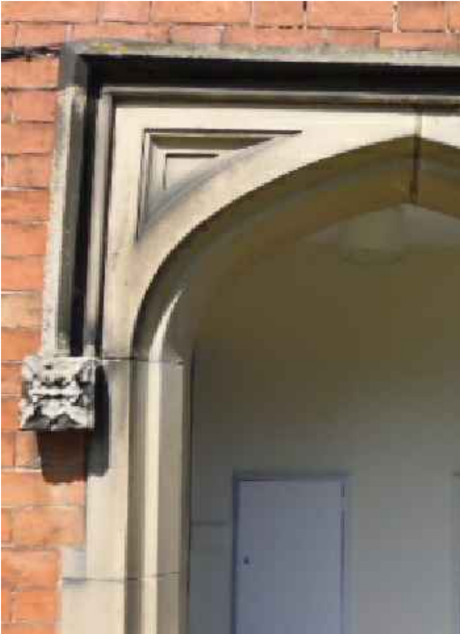
Photo 5 - Typical Stone Lobby Detail
