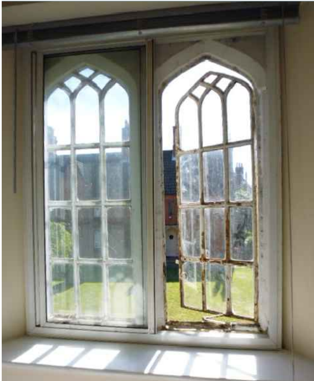
Internal Photo Of Cast Iron Period Window And Existing Secondary Glazing.
