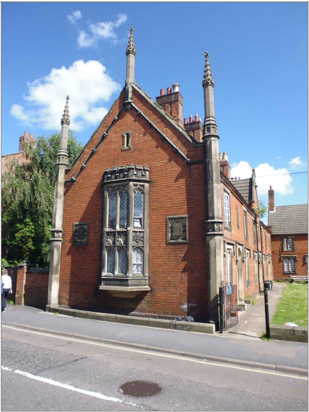
External Photo Of Cast Iron Period Window And Leaded Light Glazing. (Windows B1 to B4)
