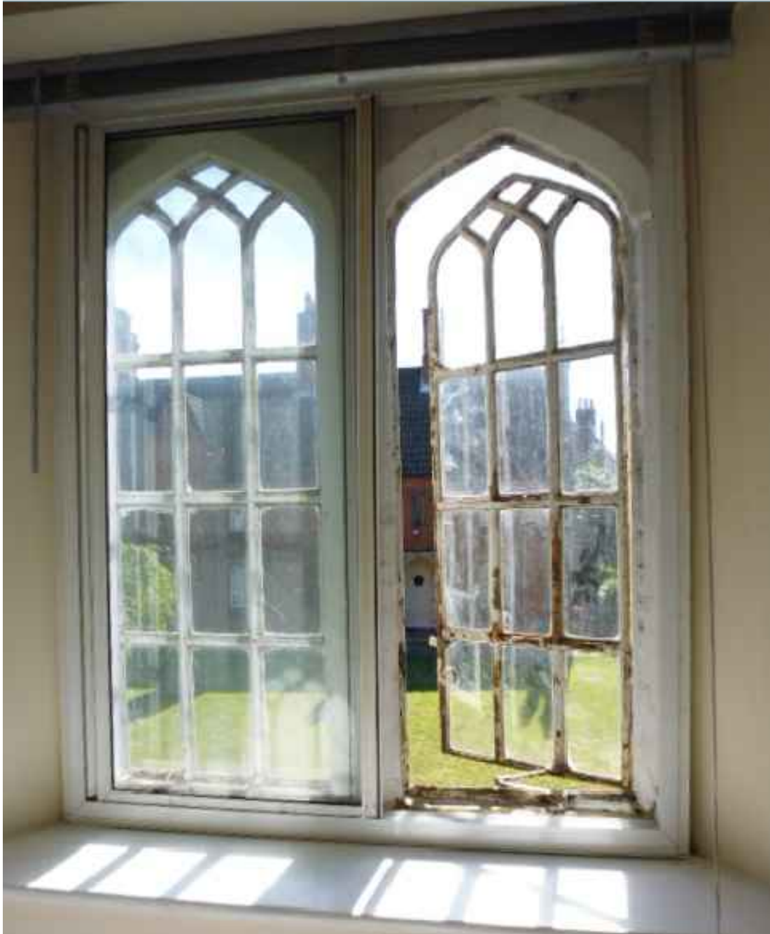
Internal Photo Of Cast Iron Period Window And Existing Secondary Glazing (Windows 1 to 35).
