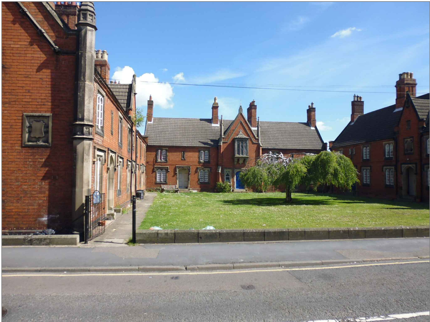
External Photo Property Elevations And Courtyard.
