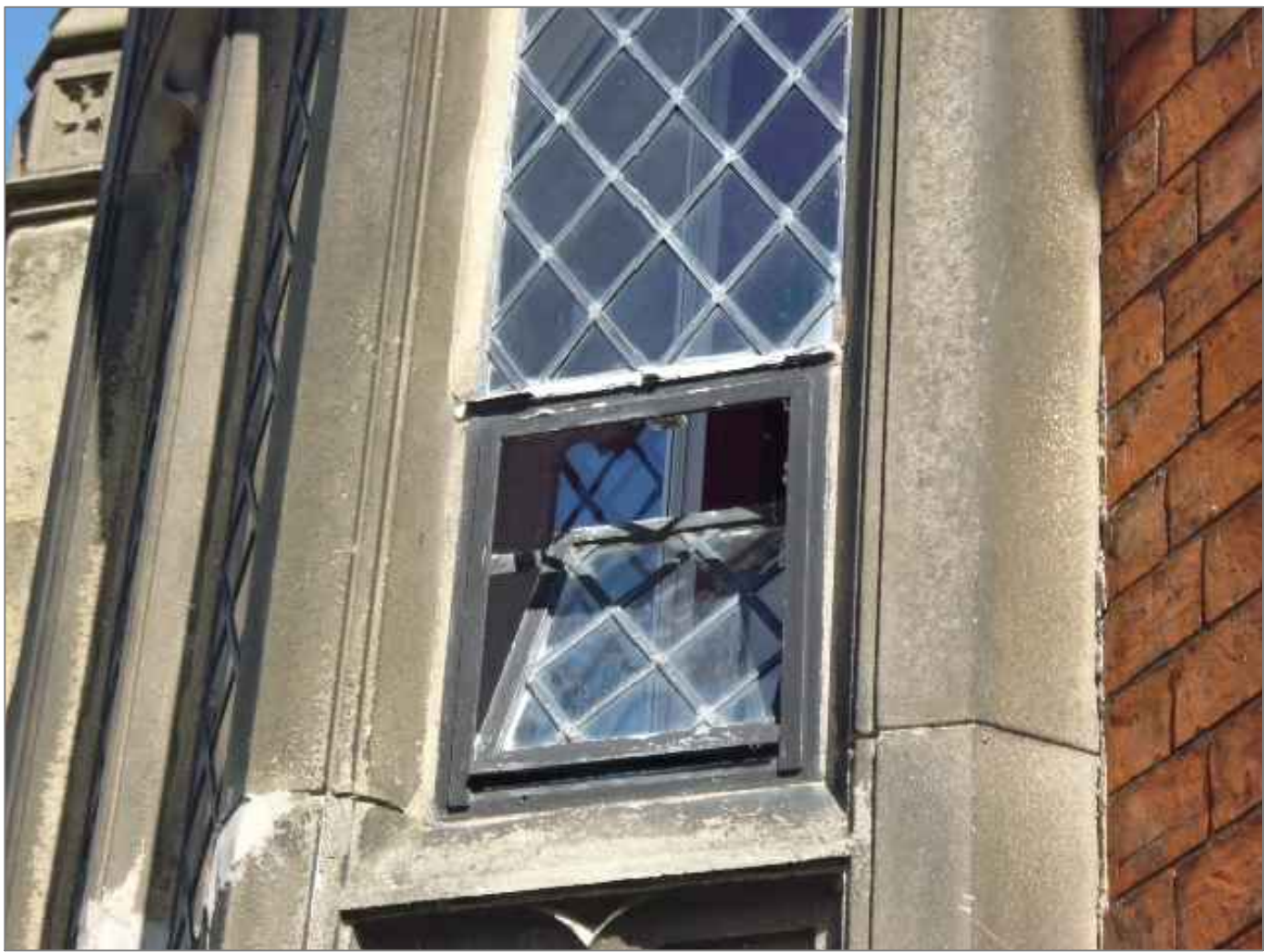
External Photo Of Cast Iron Period Window And Leaded Light Glazing. (Windows B1 to B4)
