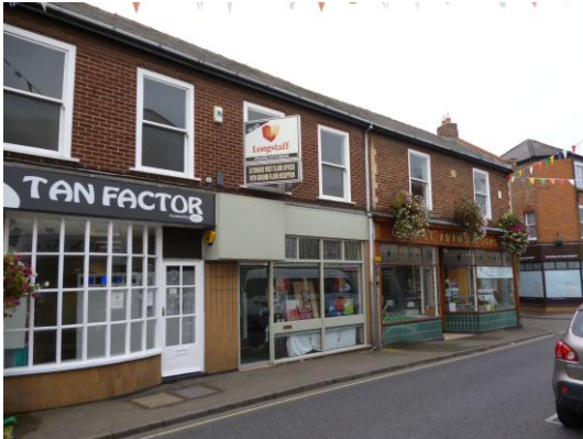
Fig. 02 – General view of Crescent frontage
