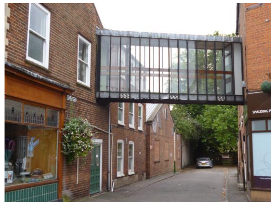
Fig. 05 – Detailed view of elevated walkway.
