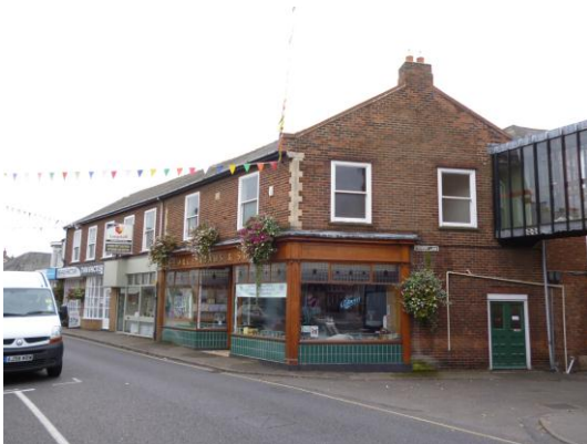
Fig. 04 – General view of elevated walkway
