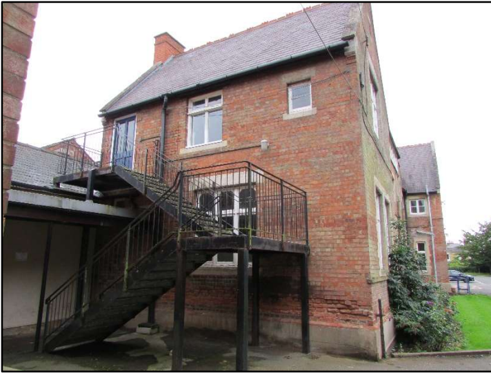
Figure 17 East end of original school building.
