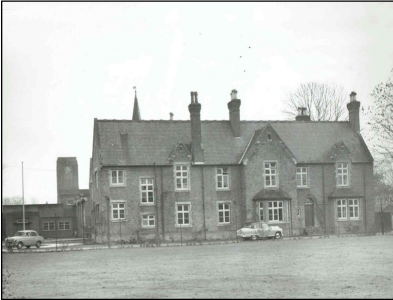
Figure 7 West elevation of old school Easter 1959 (School photograph album).
