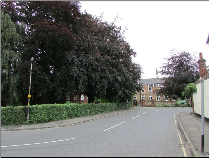
Figure 19 View south along Haverfield Road.
