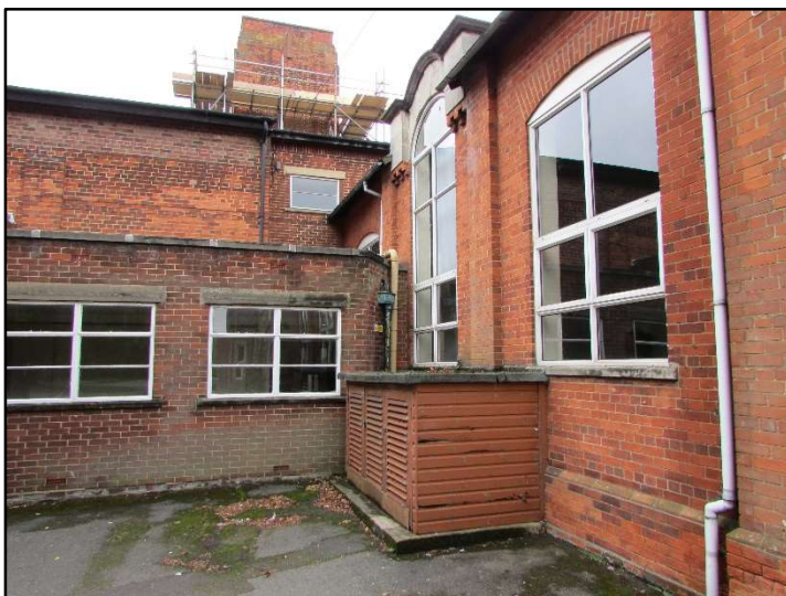
Figure 16 Junction of history block with 1930s corridor.
