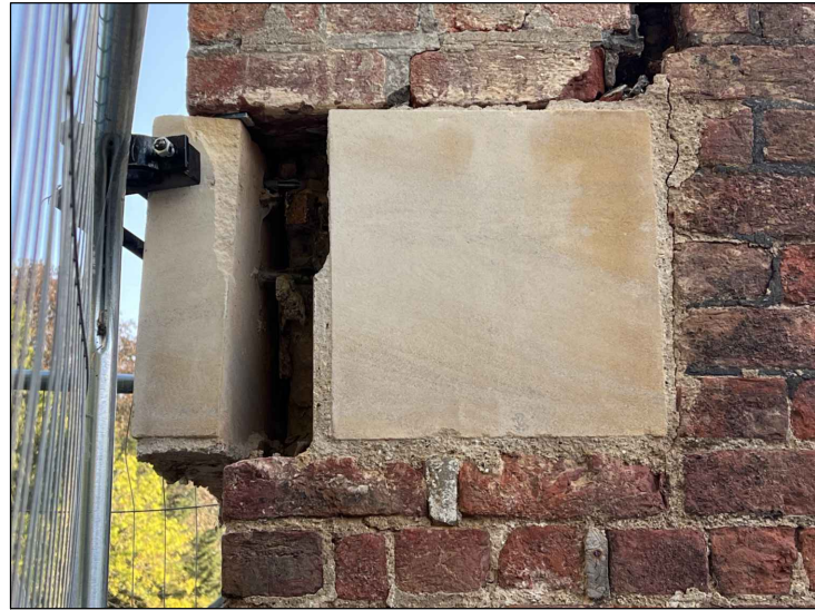
Detailed view Hinge stone displacement.
