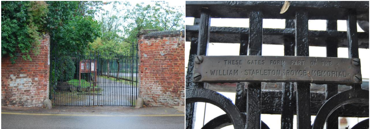
Fig 8. Photographs of the existing opening and gates with memorial plaque before being damaged
