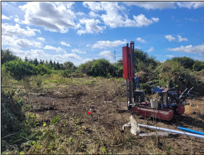
Photo 9 - Window Sampler Drilling.
