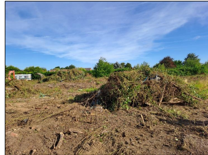
Photo 8 - Overlooking Northern Central Area of Site.
