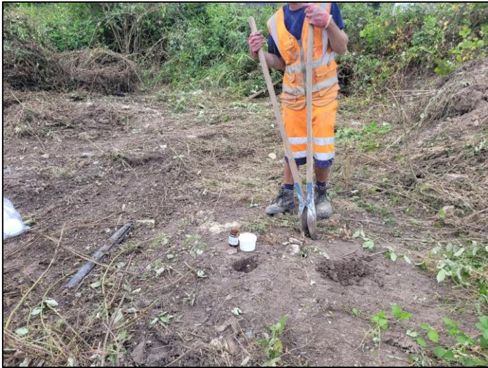
Photo 11 - Excavation of HTP.
