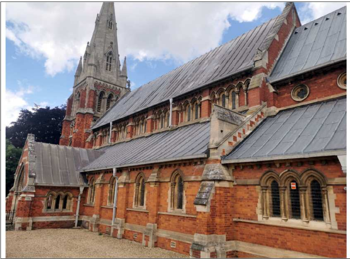
Plate 9) southern elevation of the Church of St Pauls (NHLE 1306702), looking north-west
