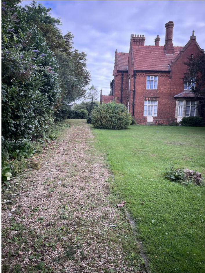
Looking north from within the site at the subject building along the existing gravel driveway
