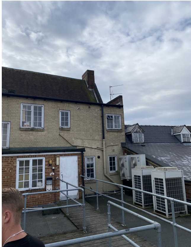
Rear of Bentley's and 1 and 2 Chapel Lane
