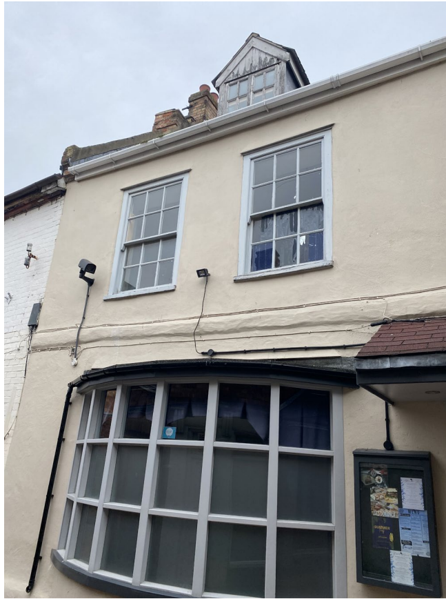
3 Chapel Lane (Grade II Listed Building)
