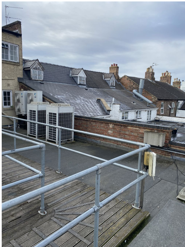
Looking across to 1-3 Chapel Lane from the rear of 2 New Road at first floor.
