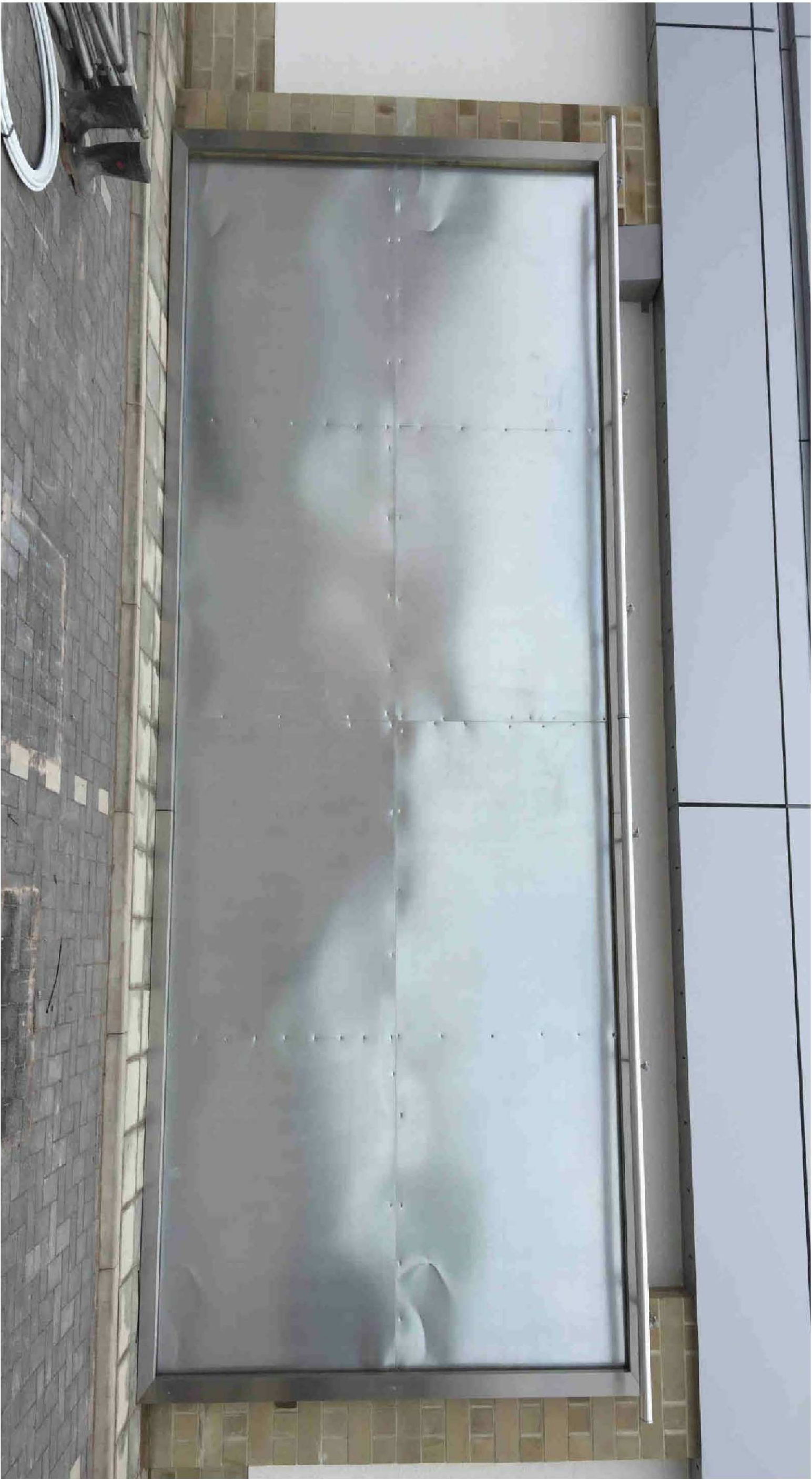
Daylight view of Typical Billboard Frame
