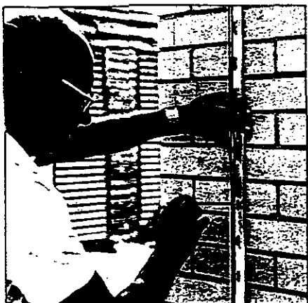
1 Plumb the Connector and mark the positions of the fixing holes ready for drilling
