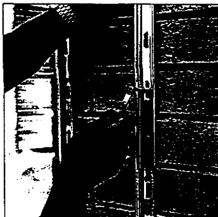
2 Fix Connector to wall using spanner and coach screws.
