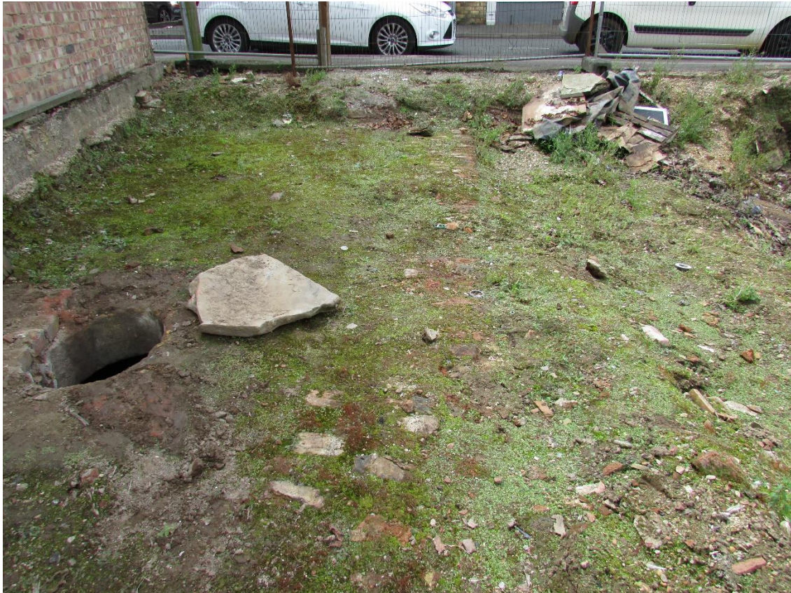
Plate 11 Manhole of Cistern on Victoria Street Site, looking west
