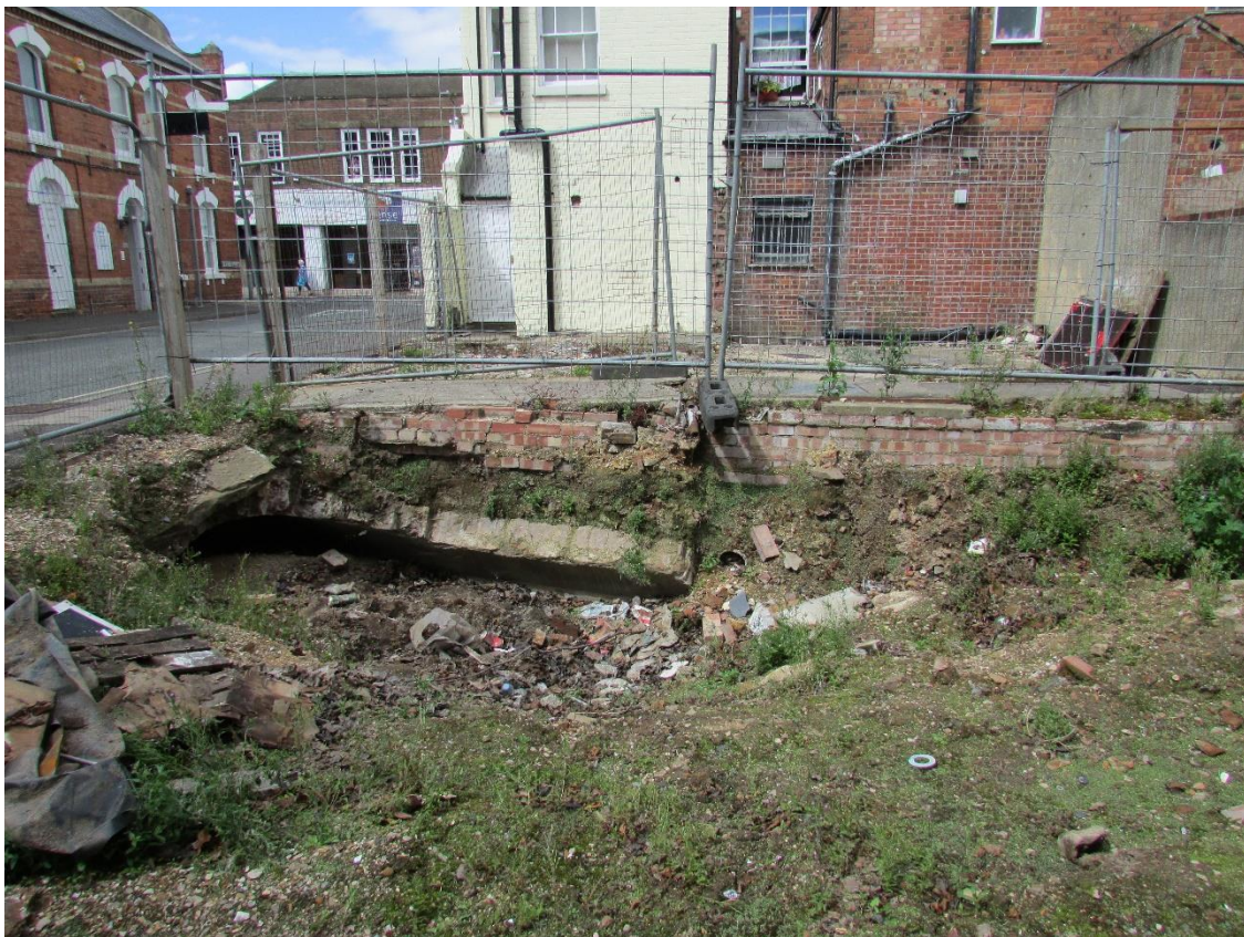
Plate 8 Remains of Cistern on Victoria Street site, looking north
