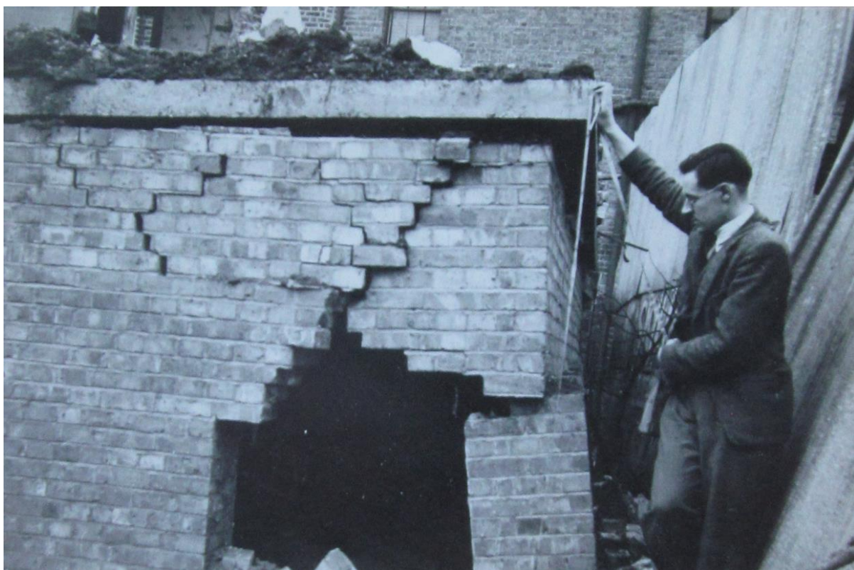
Historical Plate 15: Bomb-damaged brick and concrete surface shelter, Camberwell, London, 1941 © The National Archives (HO 186/2244)
