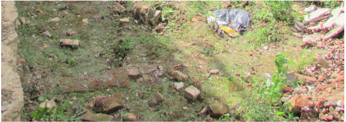
Plate 3 Detail of Plate 2 north-south brick wall, looking west
