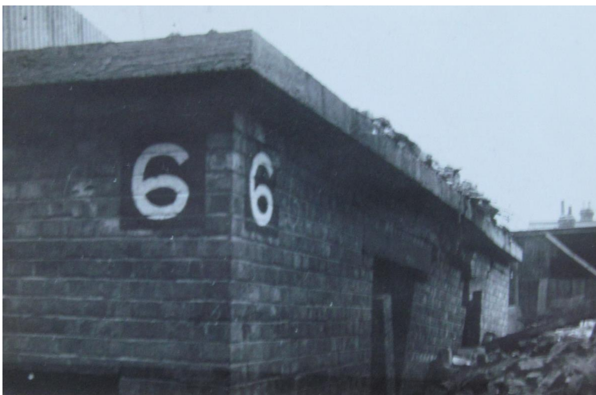
Historical Plate 16: Slightly bomb-damaged brick and concrete surface shelter, Camberwell, London, 1941 © The National Archives (HO 186/2244)
