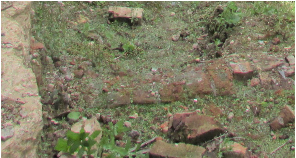
Plate 4 Detail of Plates 2 and 3 north-south brick wall, looking west
