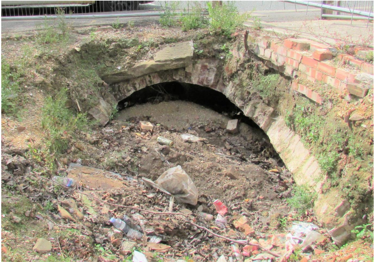
Plate 7 Detail of Plate 6 Remains of Cistern on Victoria Street site, looking west
