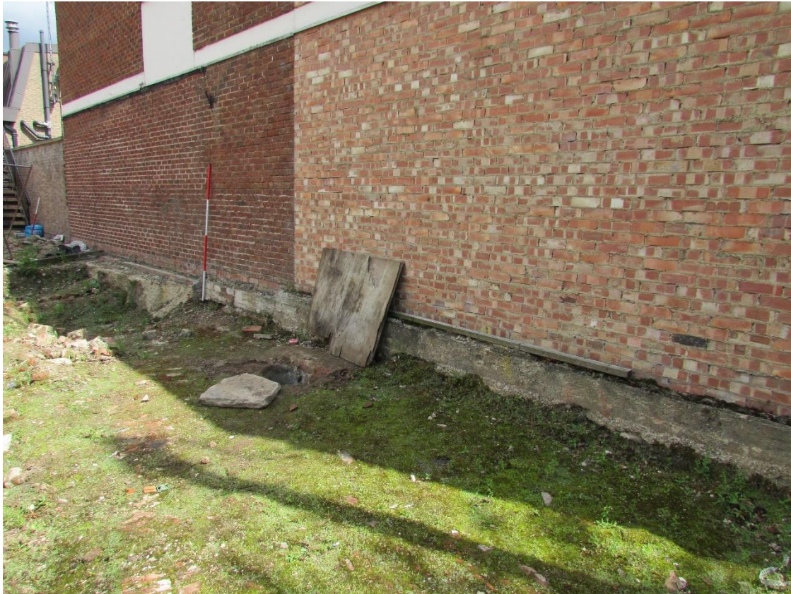
Plate 15 Victoria Street site showing Library wall looking east
