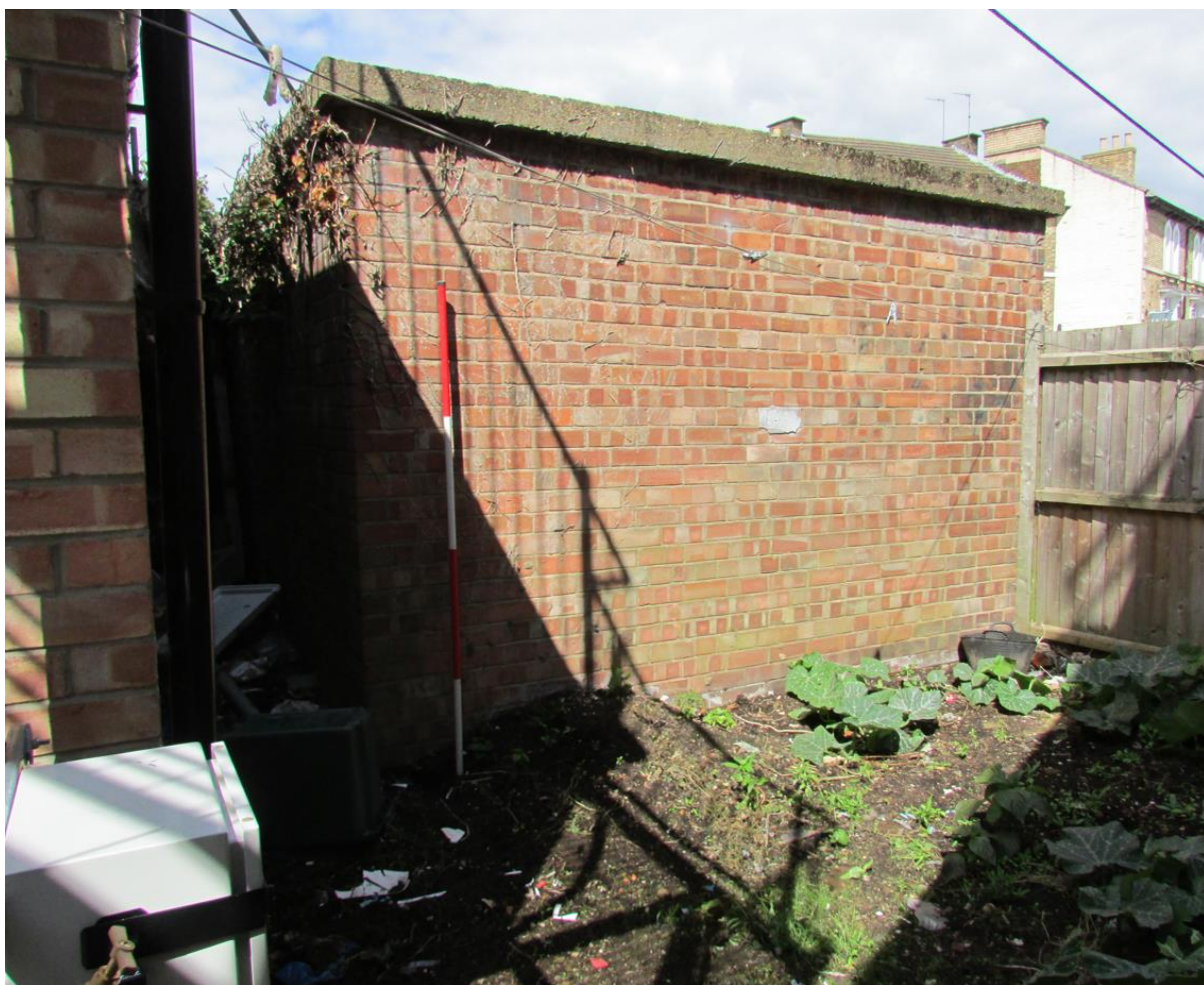
Plate 47: South elevation of the shelter, looking northeast IMG_2374
