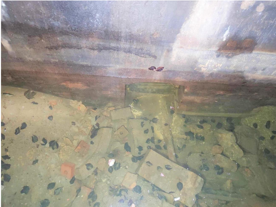
Plate 23 South wall & east drain in Cistern on Victoria Street Site, looking south from manhole
