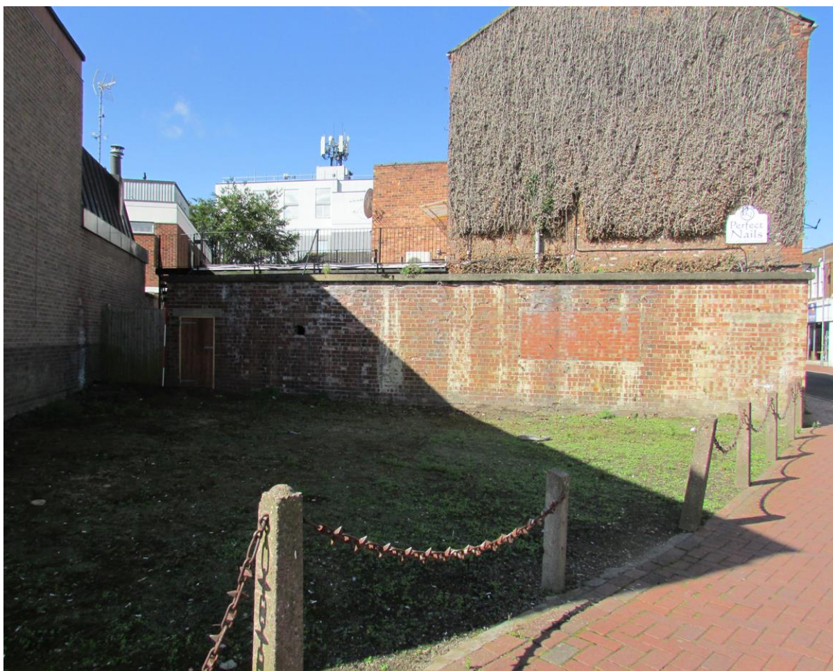
Plate 37: East elevation of the air raid shelter, looking southwest, showing northwest wall of former bank (left) and east wall of no. 19 Station Street (right). This photograph was taken in August 2023 after the southern entrance had been reopened IMG_2300
