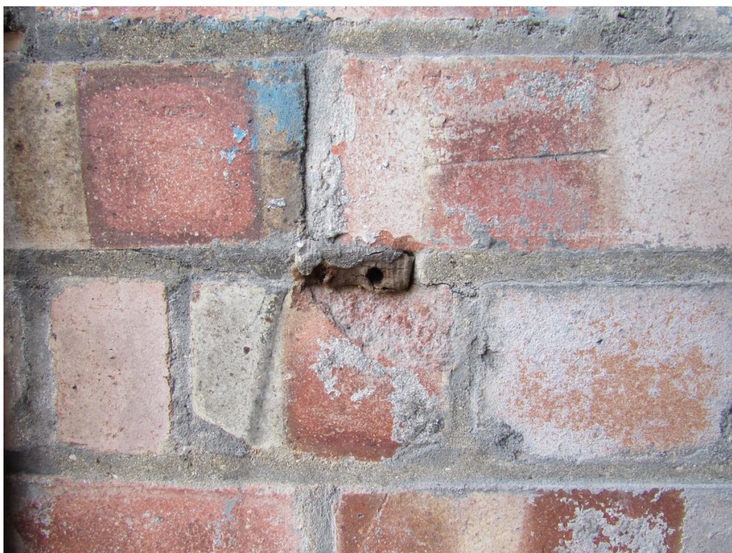
Plate 51: Close-up view of attachment point for possible doorframe in wall of outer south entrance IMG_2323
