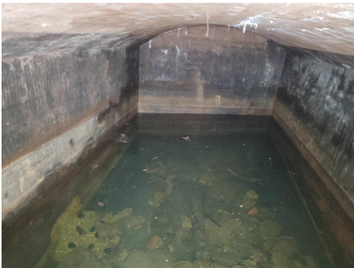
Plate 21 Cistern on Victoria Street Site, looking west from the manhole
