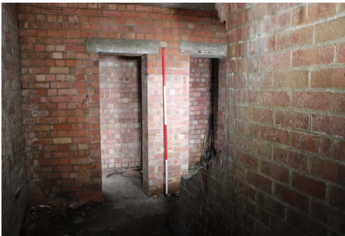
Plate 56: Interior view of inner (south) entrance (left), partially demolished central partition wall (nearest to camera) and south cubicle IMG_1510
