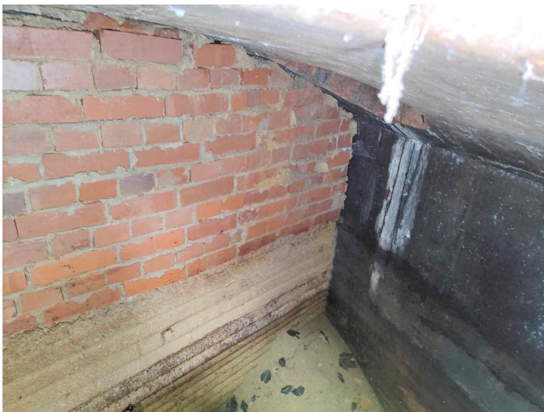
Plate 26 East blocking wall and south wall in Cistern on Victoria Street Site, looking south-east from manhole
