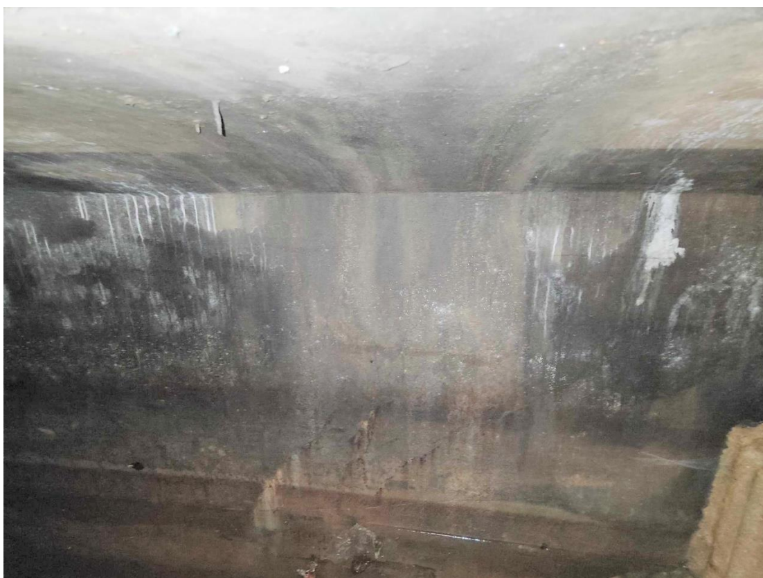
Plate 31 North wall in Cistern on Victoria Street Site, looking north from manhole
