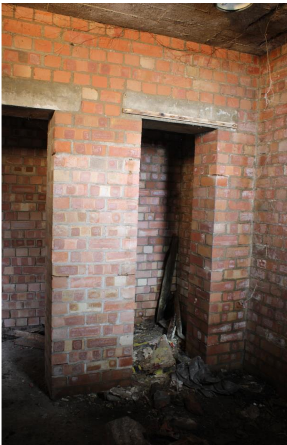
Plate 58: Inner (south) entrance (left) and entrance to south cubicle (right), looking southwest IMG_1581
