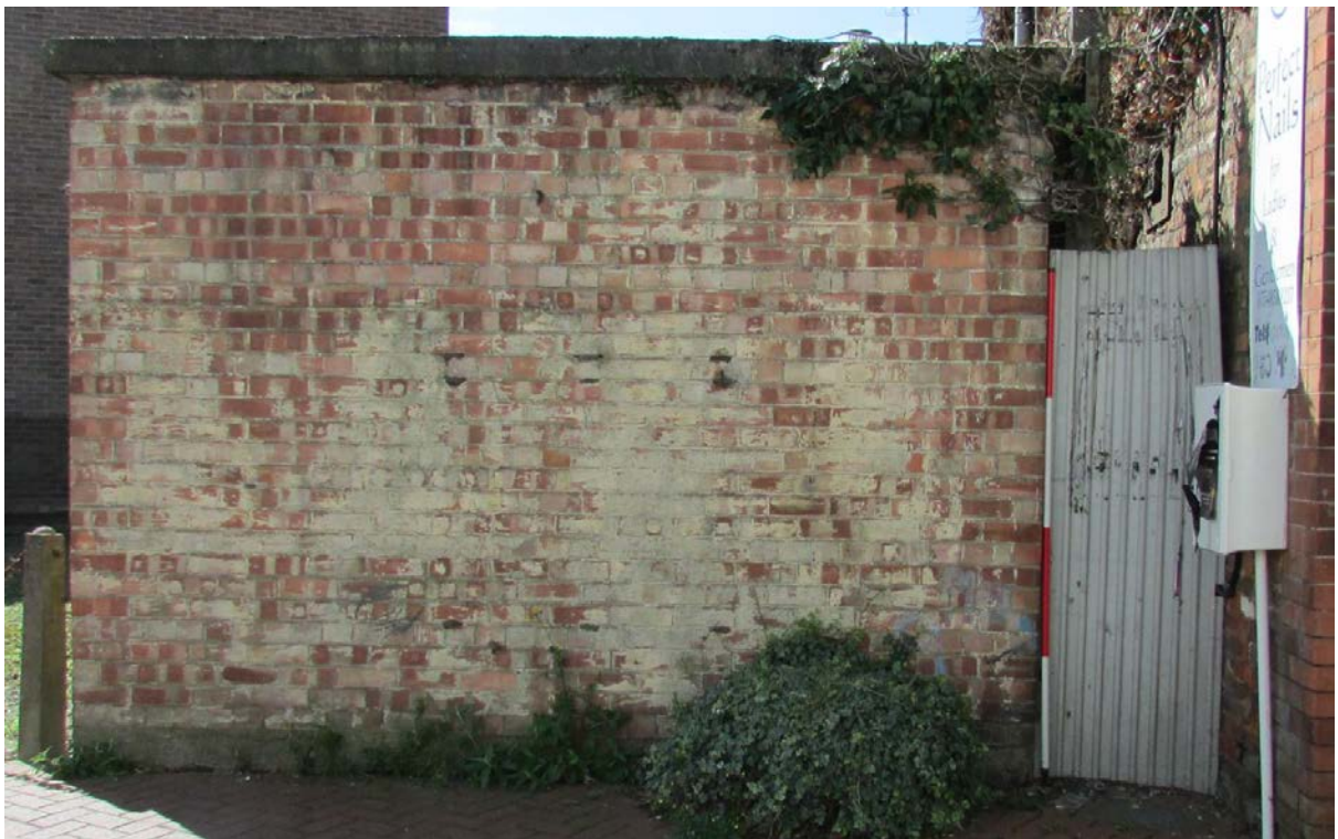
Plate 44: North elevation of the shelter, looking south IMG_2312
