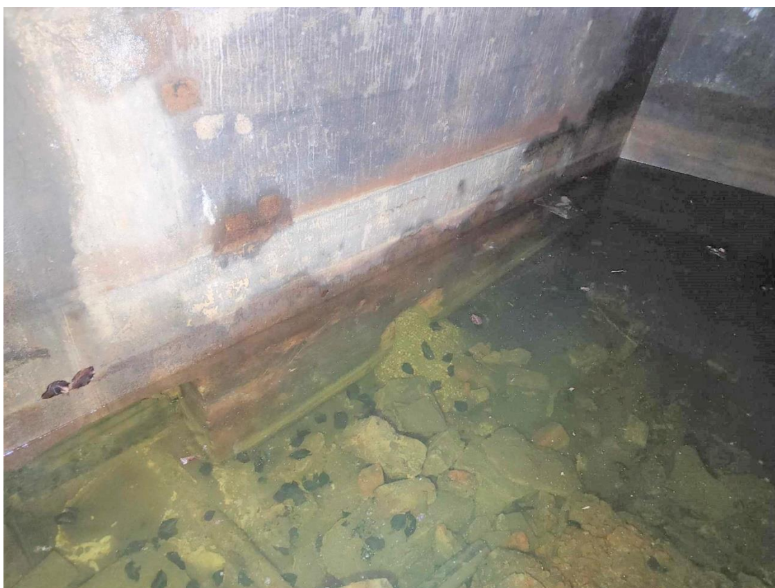
Plate 22 South wall & two drains in Cistern on Victoria Street Site, looking south-west from manhole
