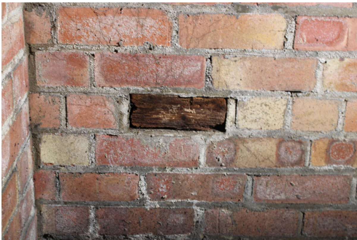
Plate 71: Timber anchor for probable bench seating in west [?] shelter compartment IMG_1578
