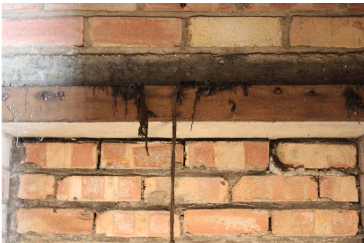
Plate 61: Remains of the gas curtain at the inner north entrance to the shelter IMG_1533
