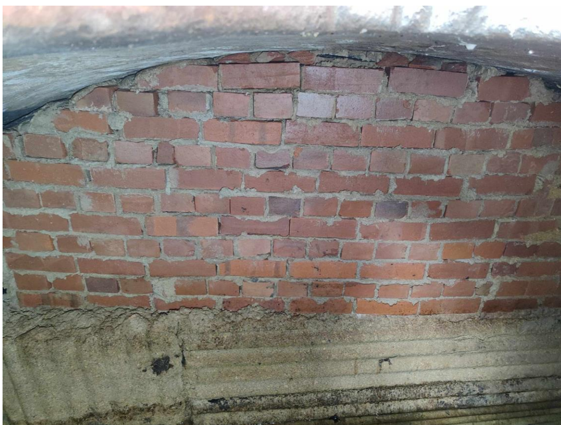
Plate 27 East blocking wall in Cistern on Victoria Street Site, looking east from manhole
