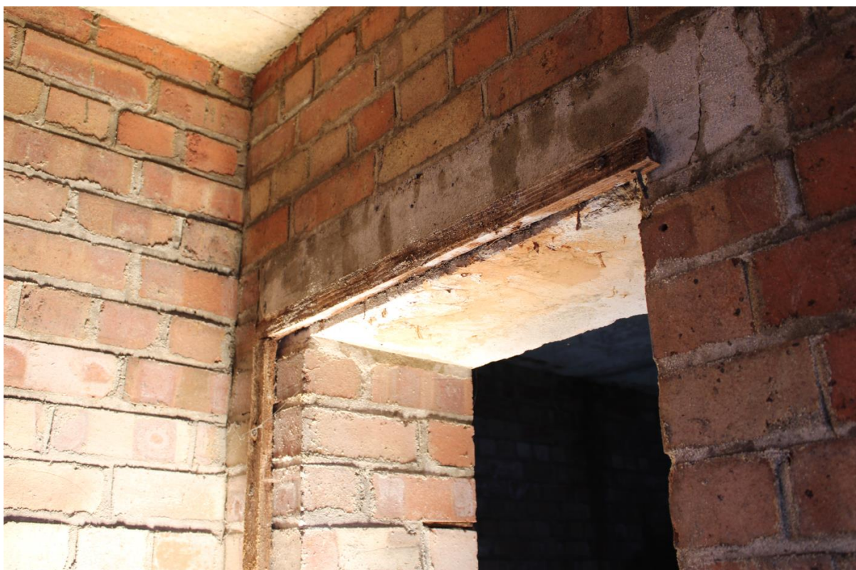
Plate 53: Close-up view of inner (south) entrance to shelter, showing incomplete simple timber frame and attachment point for probable gas curtain IMG_1607
