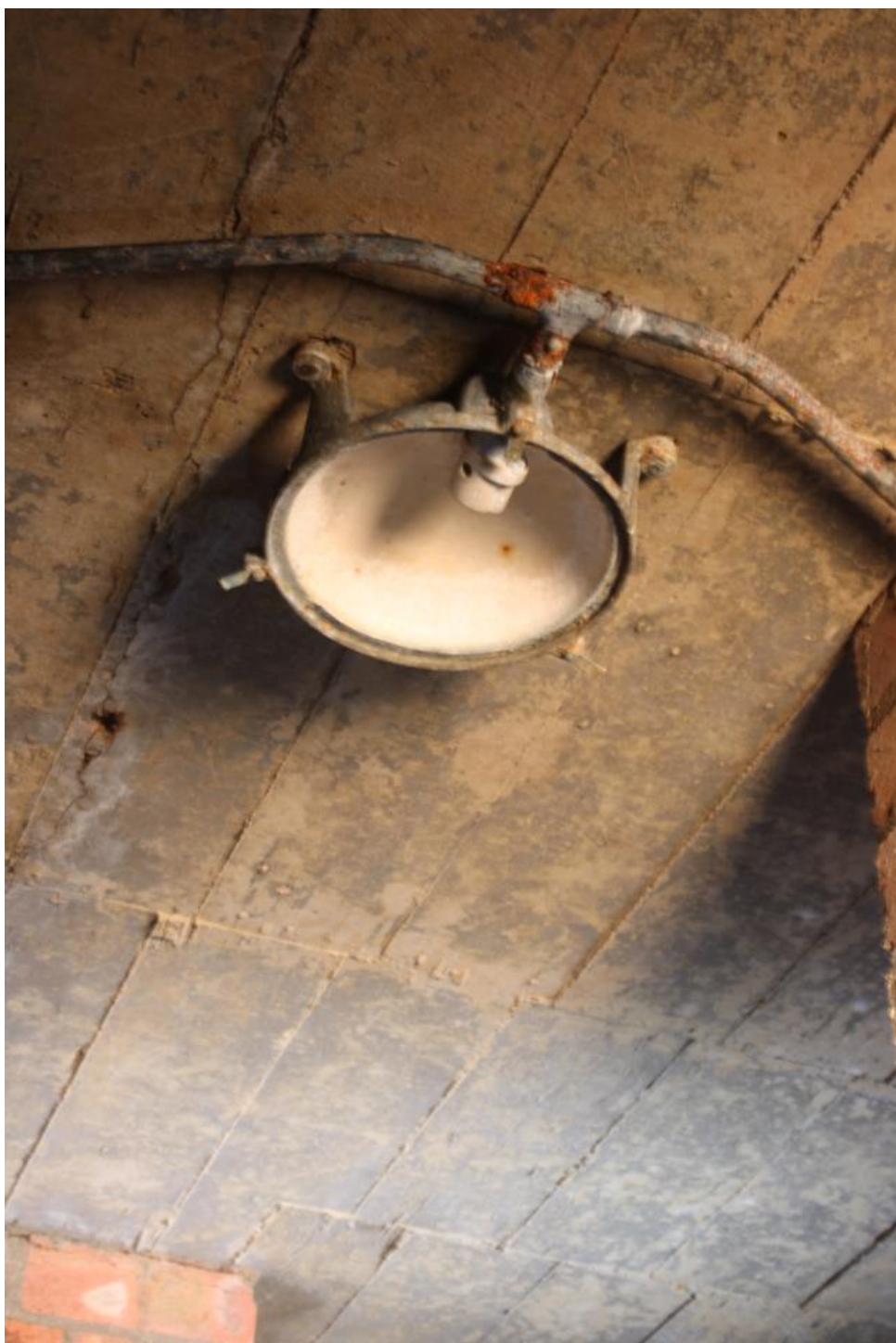
Plate 67: Detail view of central ceiling light fitting, showing method of attachment to roof slab IMG_1571
