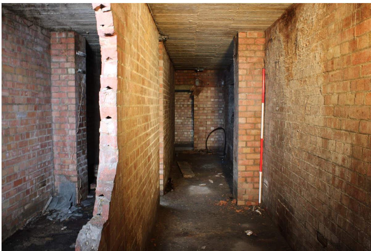
Plate 54: View of the interior of the shelter, showing central partition wall and compartments on either side, looking north towards the inner (north) entrance IMG_1498)
