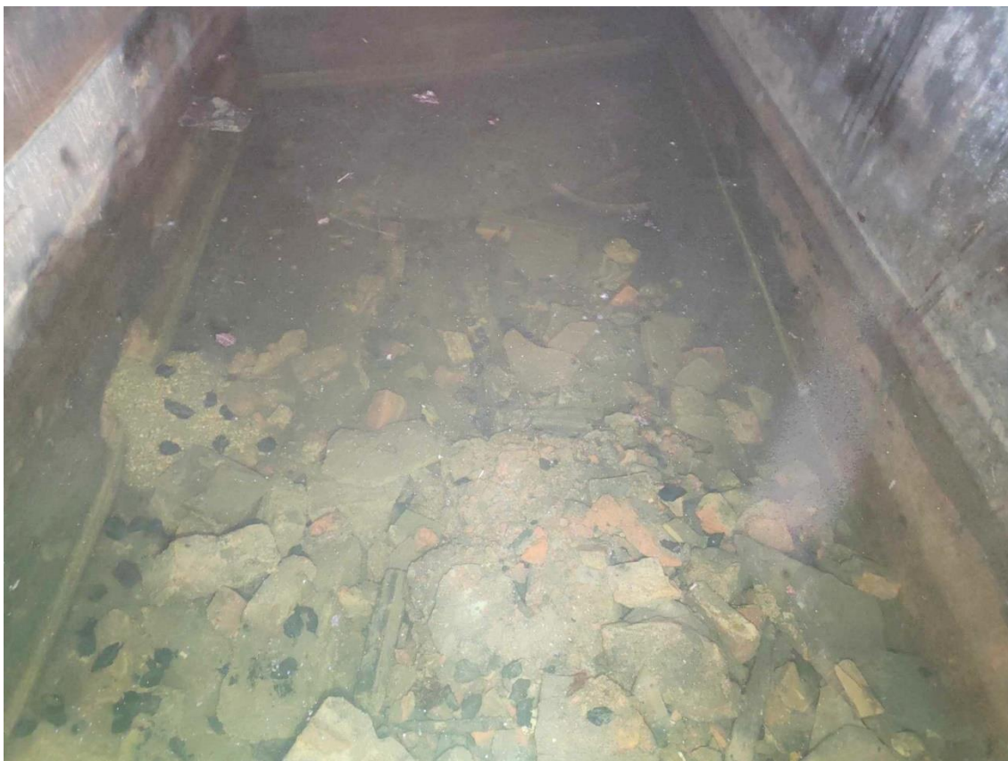
Plate 33 Rubble within the Cistern on Victoria Street Site, looking down and west from manhole
