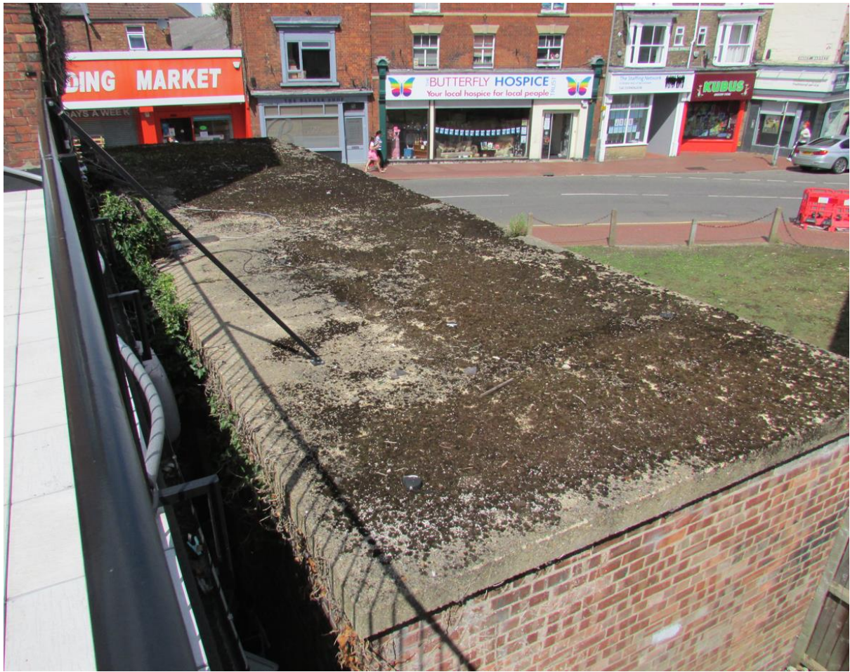
Plate 48: Concrete roof slab of the shelter, looking northeast from no. 19 Station Street flat IMG_2377
