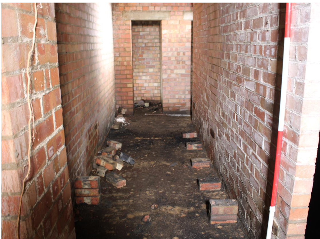
Plate 70: Brick supports for bench seating on the floor of west shelter compartment, north end IMG_1520
