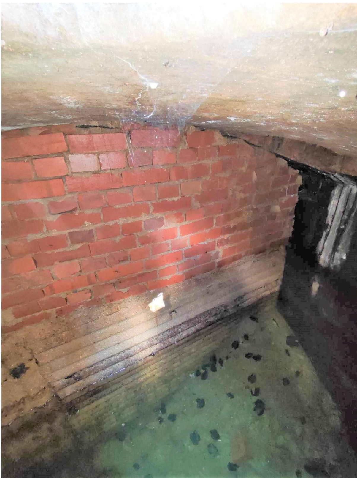
Plate 25 East blocking brick wall and south wall in Cistern on Victoria Street Site, looking south-east from manhole
