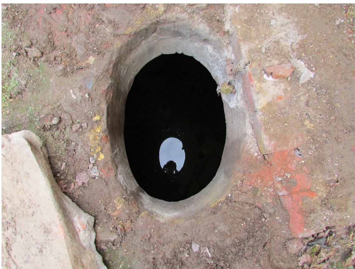
Plate 18 Manhole of Cistern on Victoria Street Site, looking down and east
