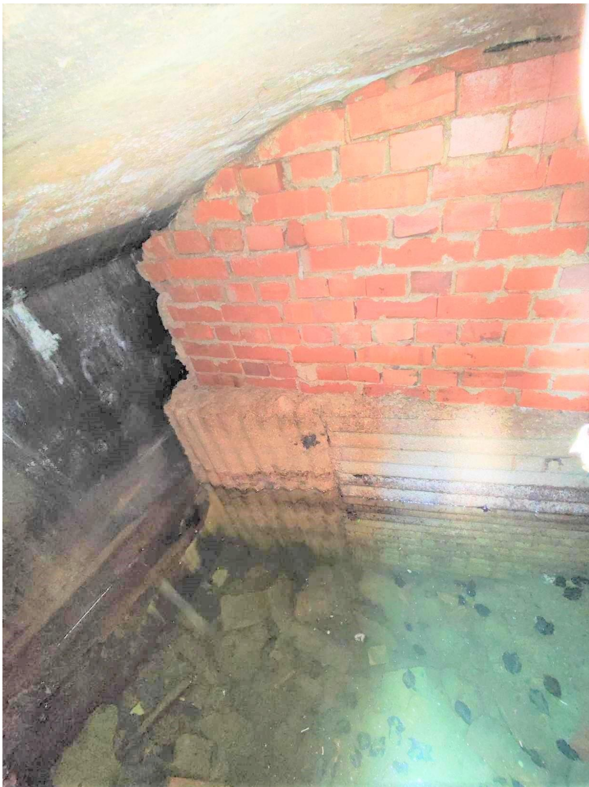
Plate 29 North wall and east blocking wall in Cistern on Victoria Street Site, looking north-east from manhole
