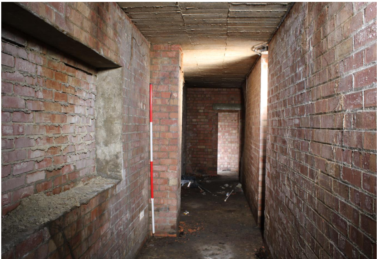
Plate 74: Infilled post-war window opening in east wall of the shelter, looking south IMG_1558
