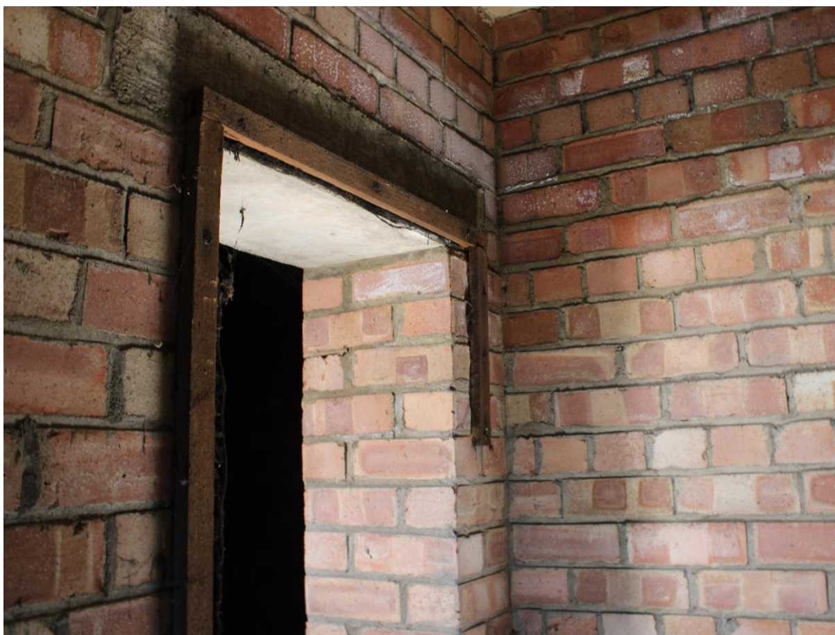
Plate 60: Timber frame attached to outer face of inner (north) entrance, looking southwest IMG_1539
