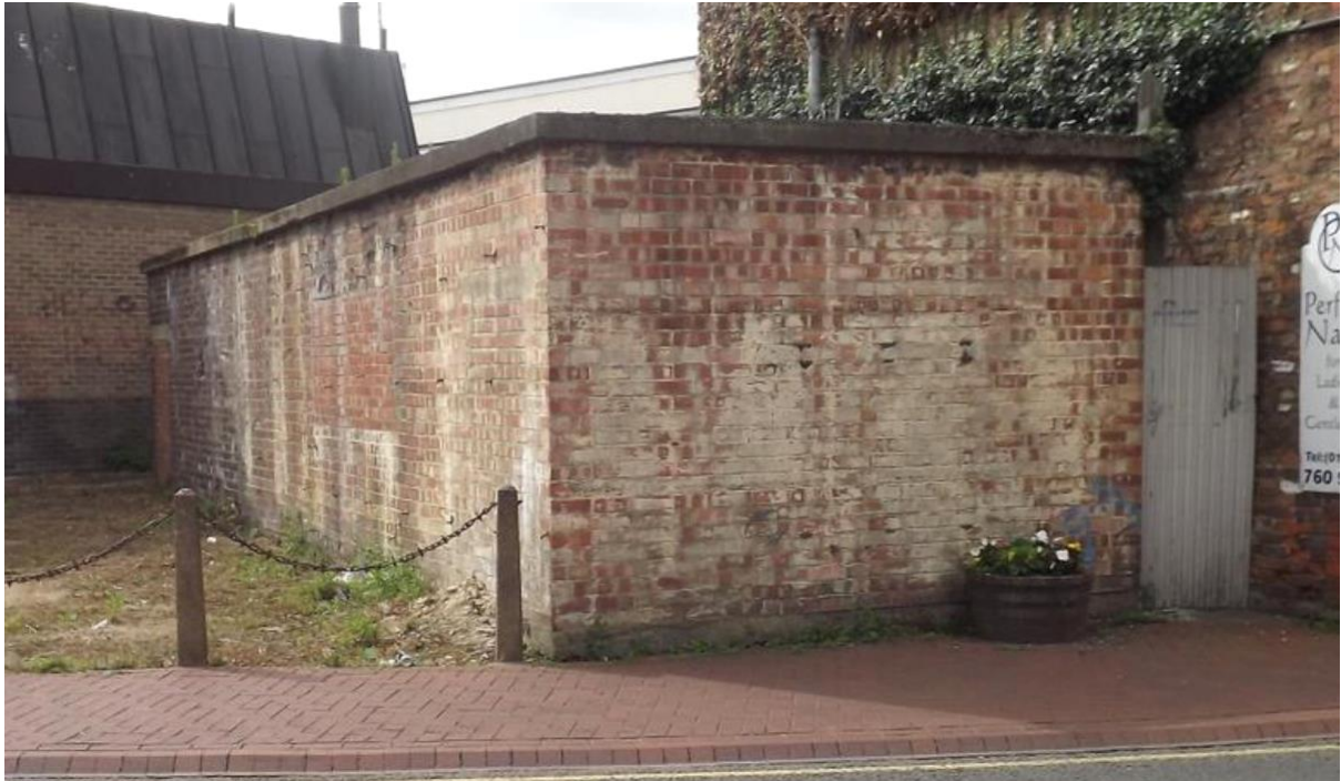
Plate 35: The air raid shelter prior to reopening, looking southwest © Stuart Banham (flickr)
