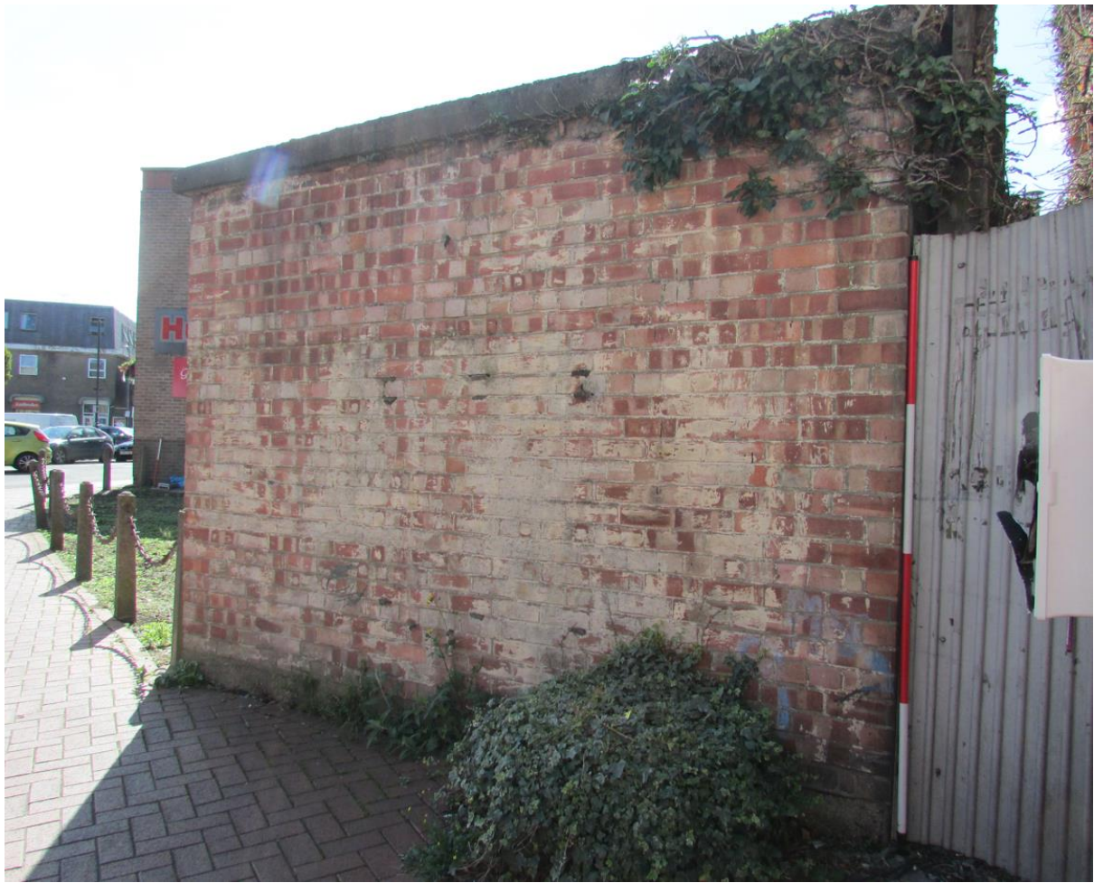
Plate 45: North elevation of the shelter, looking southeast, showing wooden pegs embedded in mortar IMG_2313
