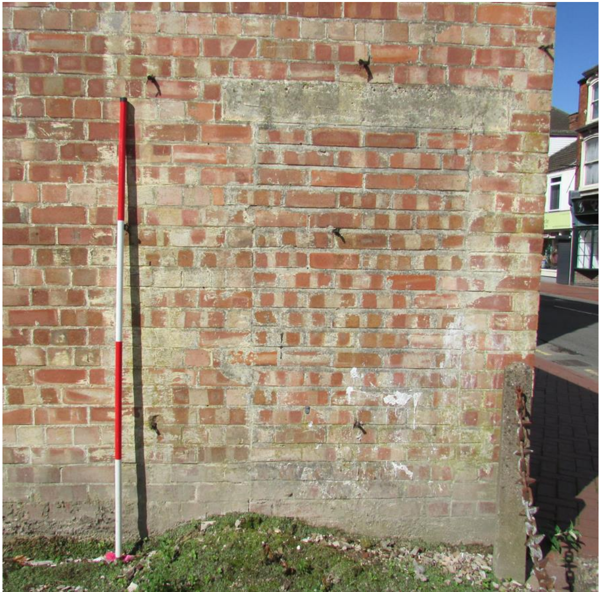
Plate 40: Bricked-in north entrance to air raid shelter, looking west IMG_2304
