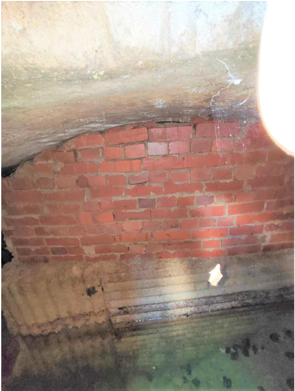
Plate 28 East blocking wall in Cistern on Victoria Street Site, looking east from manhole
