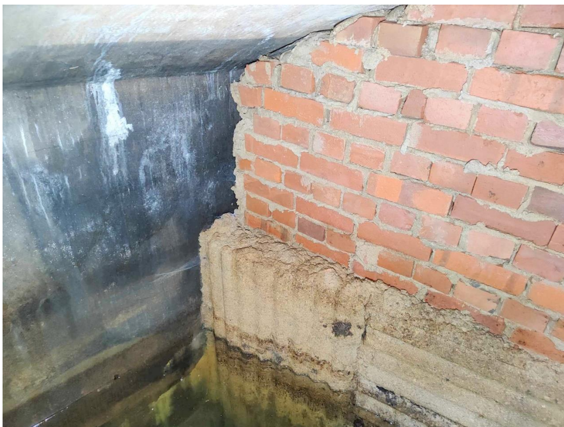
Plate 30 North wall and east blocking wall in Cistern on Victoria Street Site, looking north-east from manhole
