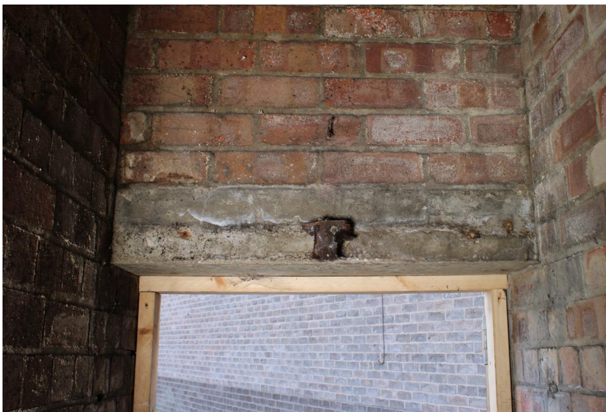
Plate 50: Rear face of concrete lintel over outer south entrance, showing wooden bracket and possible imprint of former timber doorframe attachment points in the brickwork below IMG_1606
