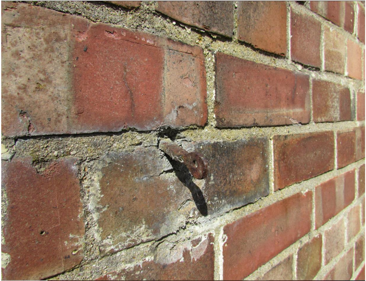
Plate 43: Metal bracket inserted into mortar in east elevation IMG_2305
