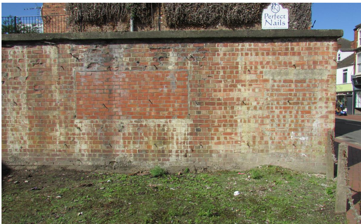
Plate 41: Aperture cut into brickwork of east elevation, infilled with post-war red brickwork, looking west IMG_2311
