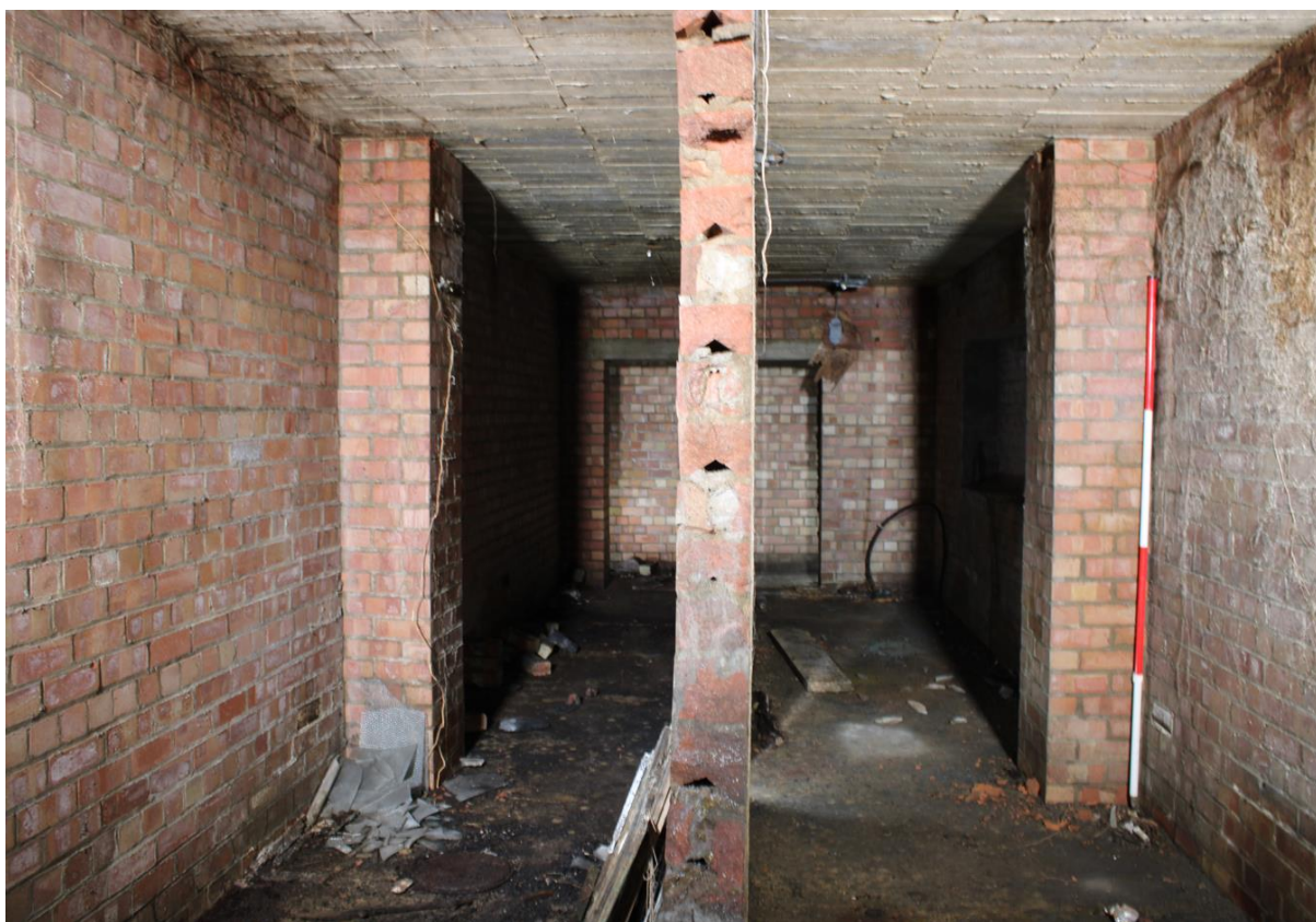
Plate 55: Another view of the interior, showing compartments on each side of central wall and north cubicle (left) inner (north) entrance (right) at the far end, looking north IMG_1501
