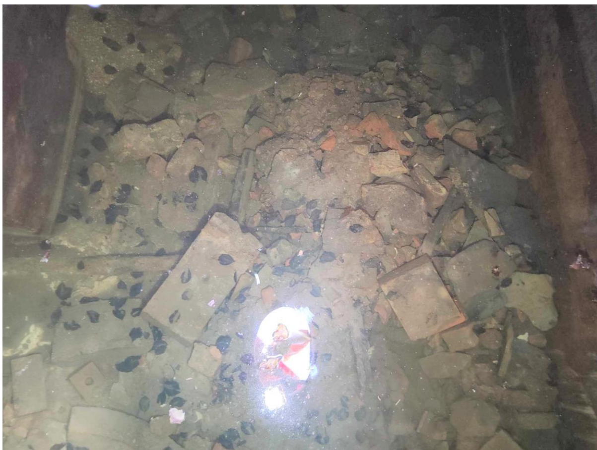
Plate 34 Rubble within the Cistern on Victoria Street Site, looking down and west from manhole
