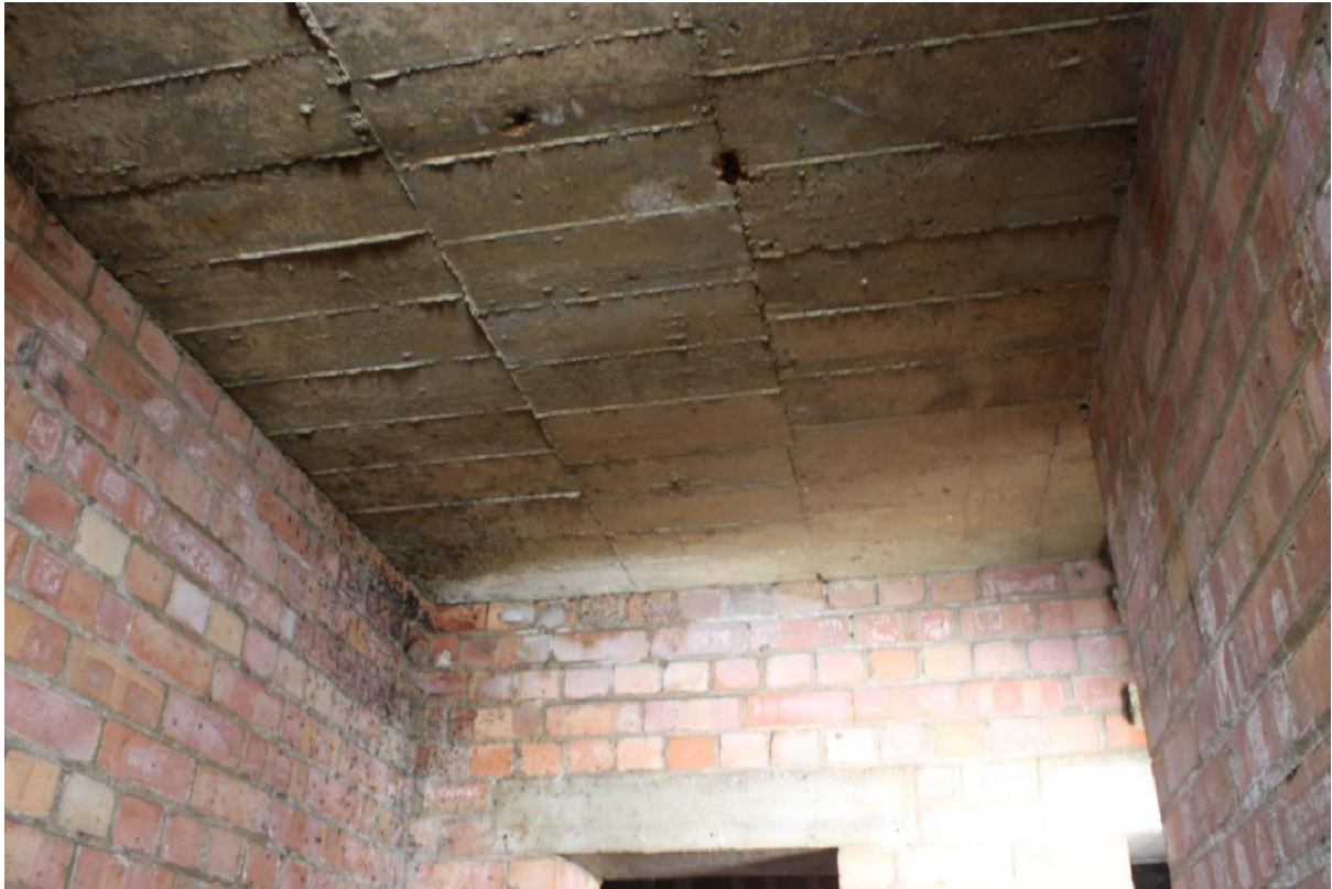
Plate 62: Imprints of timber shuttering in the concrete roof slab IMG_1528
