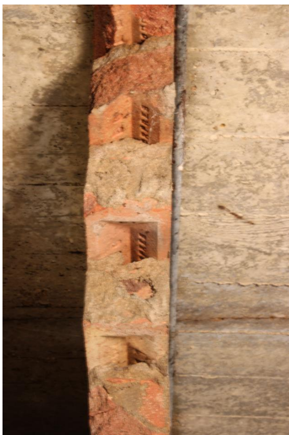
Plate 57: Detail view showing LBC 'PHORPRES' Fletton bricks used in the construction of the central partition wall IMG_1592
