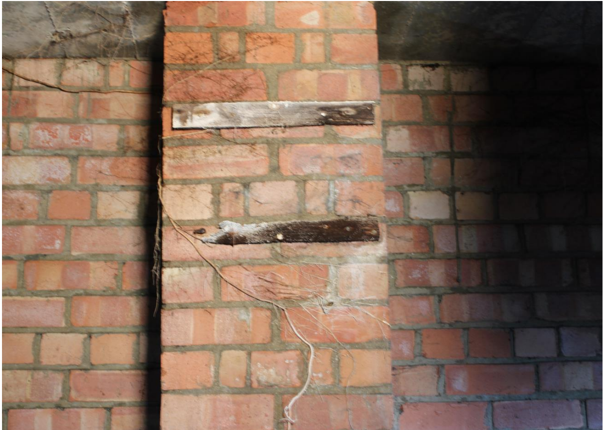
Plate 73: Timber battens attached to central brick pier in west shelter compartment IMG_1577
