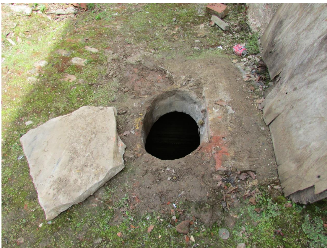
Plate 17 Manhole of Cistern on Victoria Street Site, looking east
