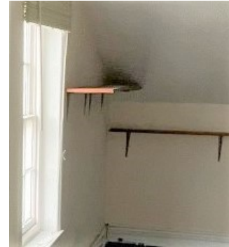
Fig 8. Modern worktops and shelves to be removed to allow installation of a bathroom
