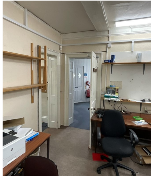
Fig 5. View of the existing office with shelving to be removed and new fire lobby to be introduced
