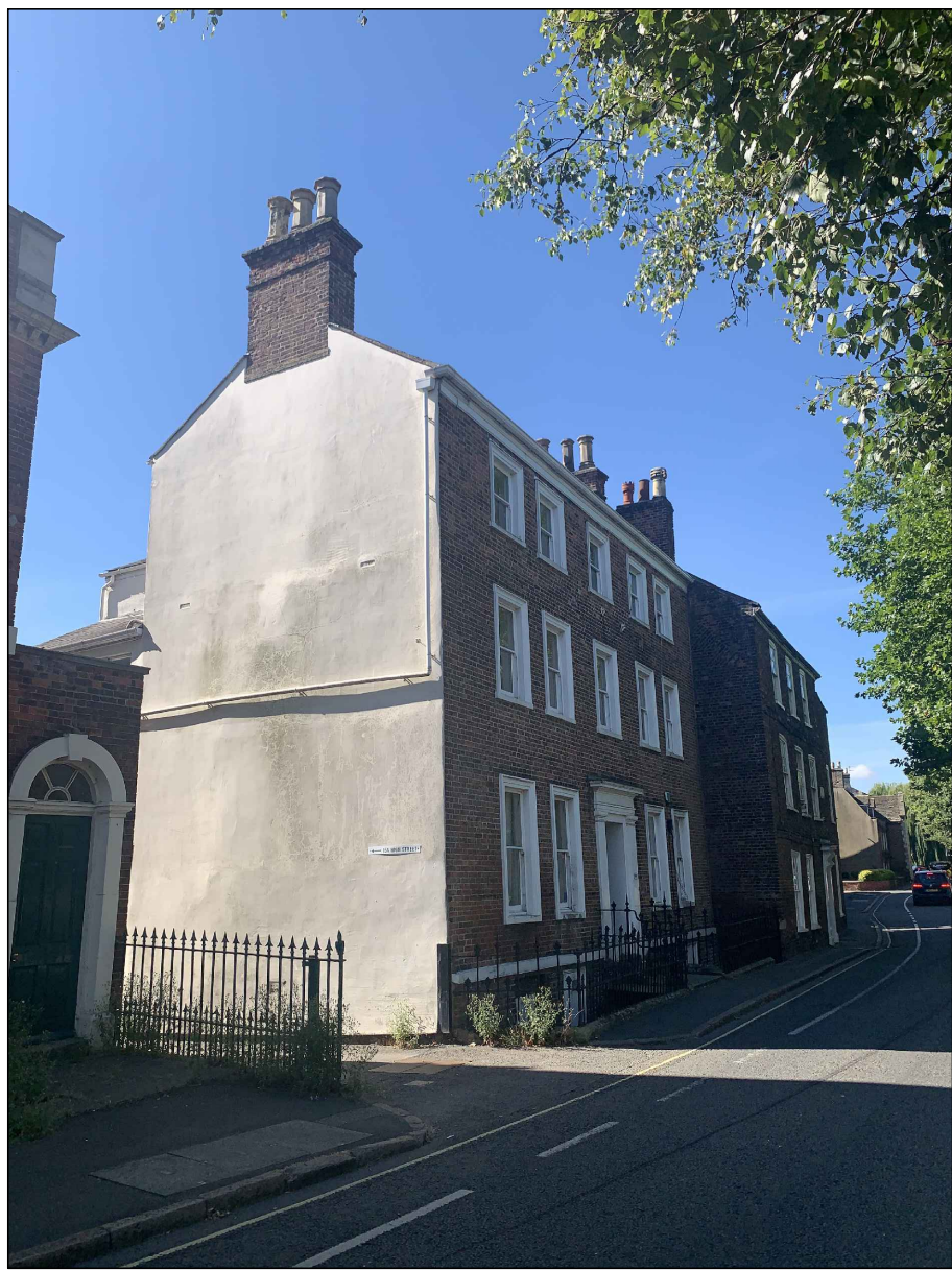
North (gable) elevation viewed from High Street
