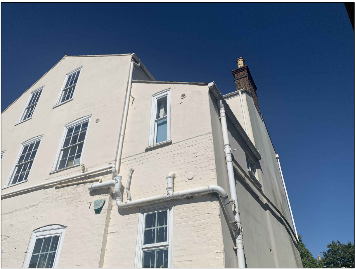
View of north-east corner of the building showing drainage that will be reconfigured.
