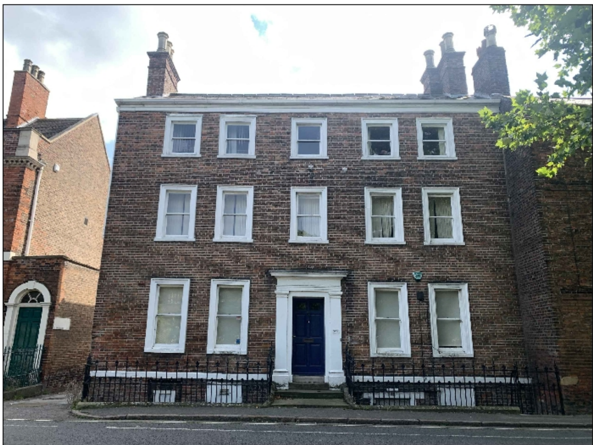
West (front) elevation viewed from the parking area
