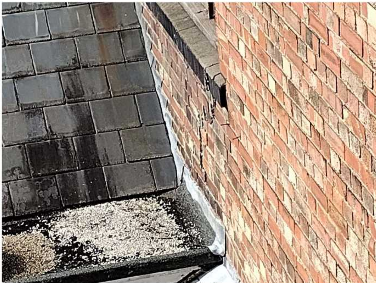
Photo 1 – Masonry Cracking below First Floor Window (South Elevation):
