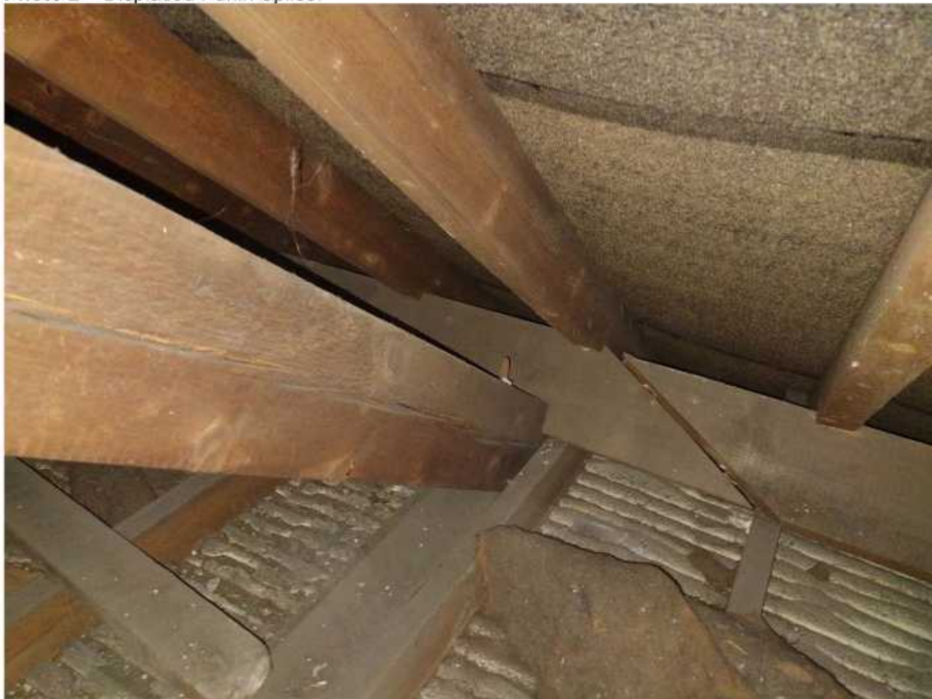
Photo 2 – Displaced Purlin Splice:
