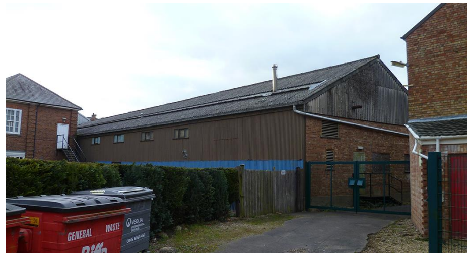
View of the rear of the site ↑
