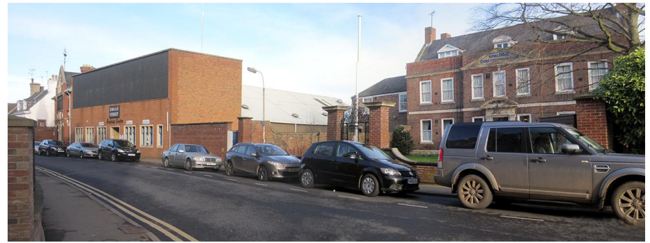
View north along Broad Street towards existing Broad Street Business Centre ↑
