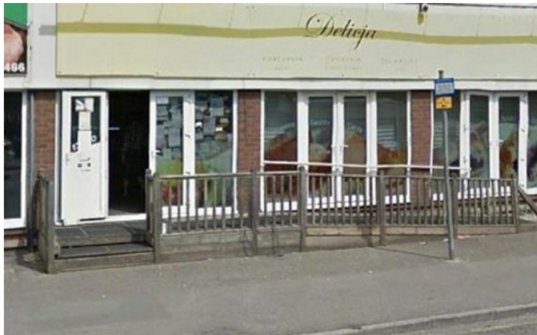
Existing Balustrade to be replaced
