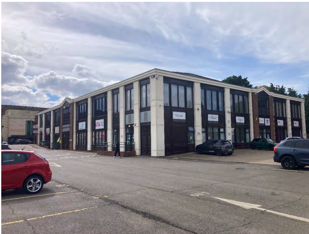
Plate 2: Broadgate House in the south-western part of the Site
