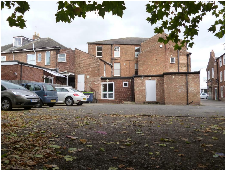
Fig. 05 – View from the rear.
