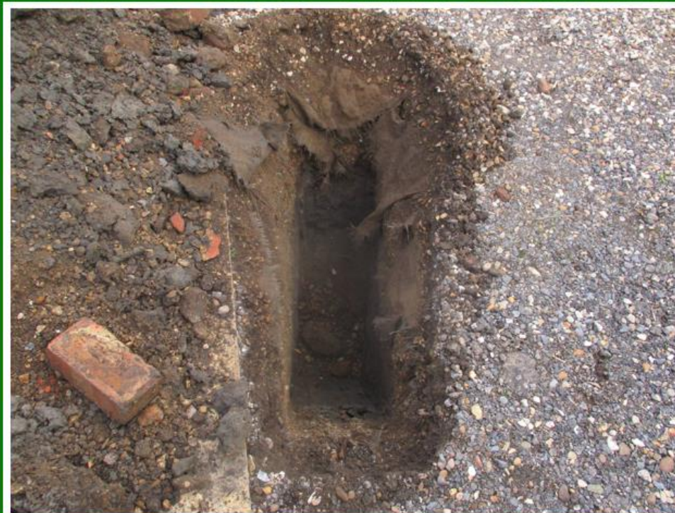
Photo No.6: TP03 pit sides and base
