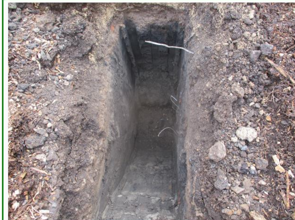
Photo No.4: TP02 pit sides and base
