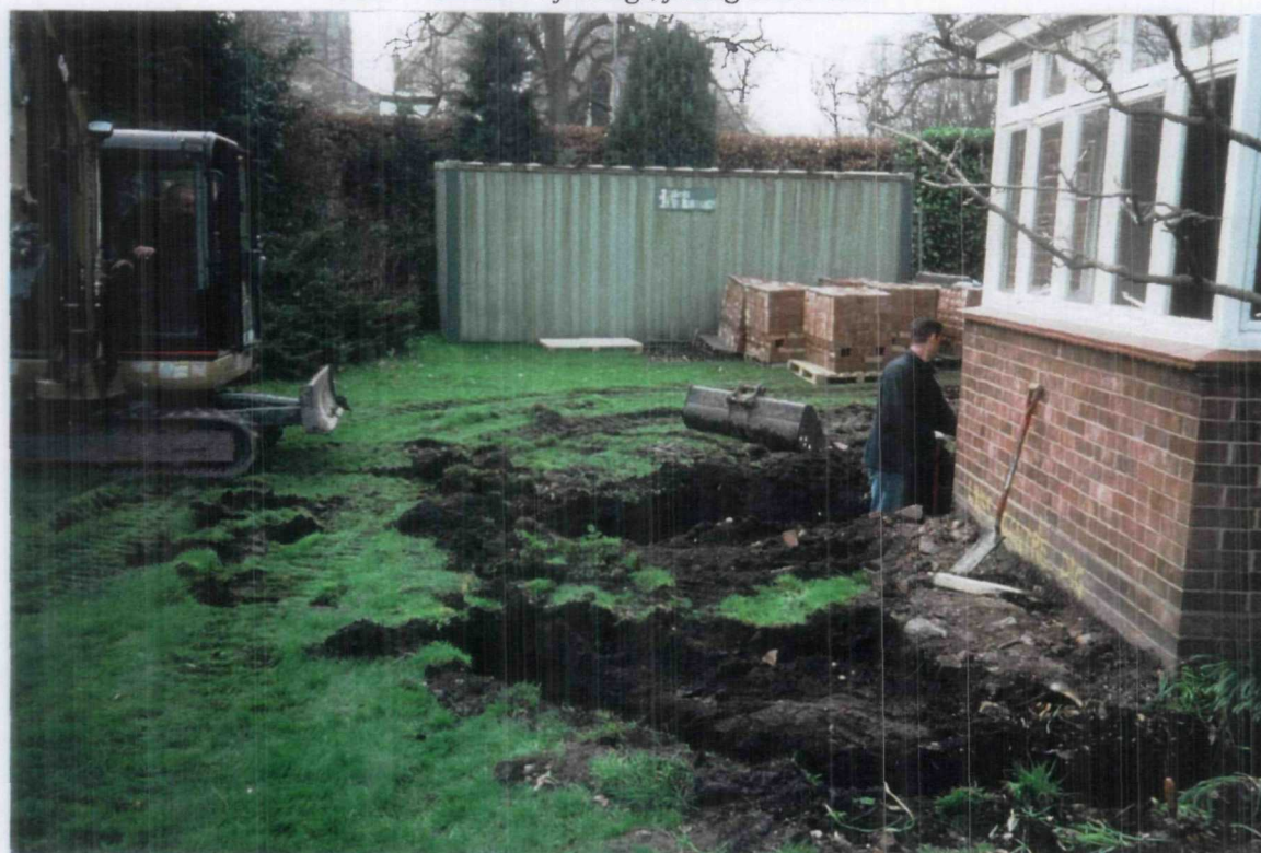
8.2.2 Conservatory footings, facing north west.
