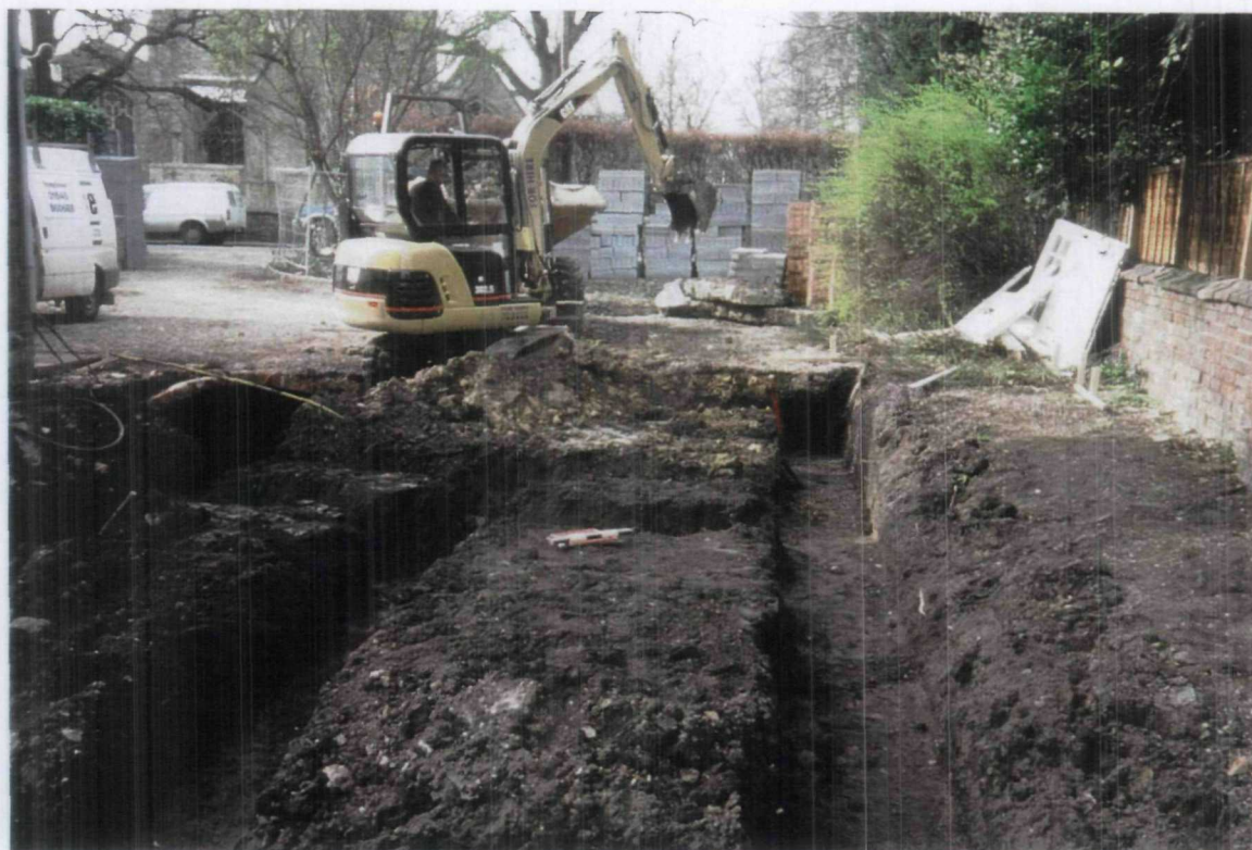
8.2.1 Extension footings, facing north west.
