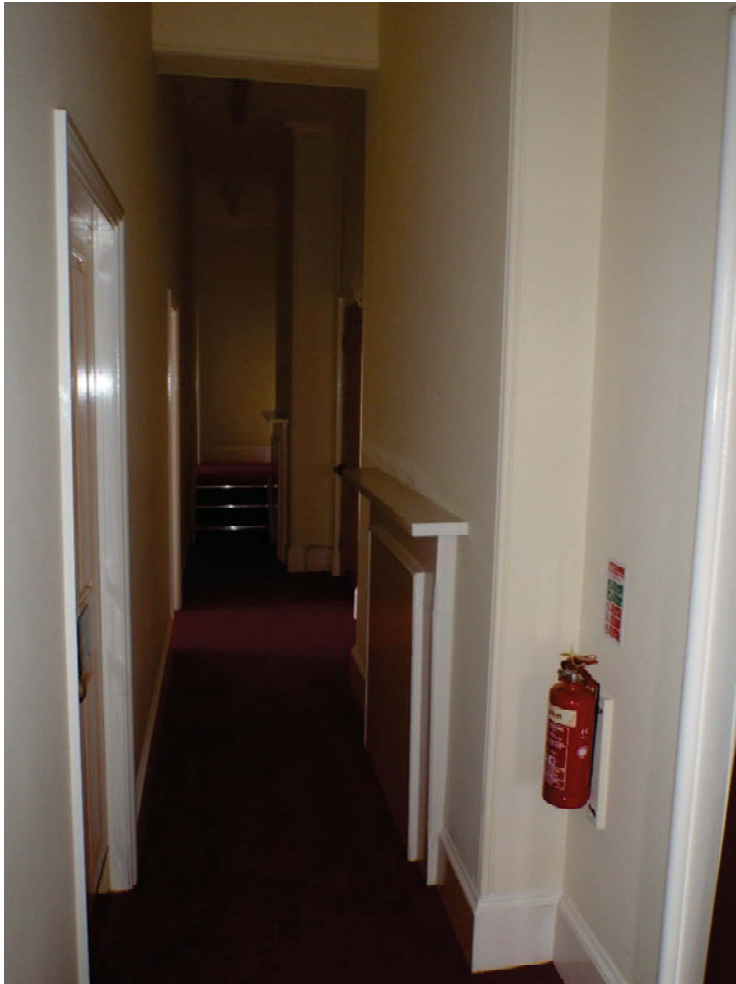
Plate 13 Corridor with interview rooms on left. Note blocked fireplaces and 'beam' of cut-through wall (top of picture)
