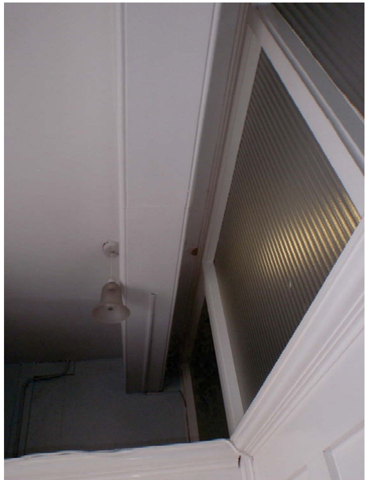
Plate 2 1 st Floor WC, panel wall with borrowed light glazing and 'beam' of cut-through wall
