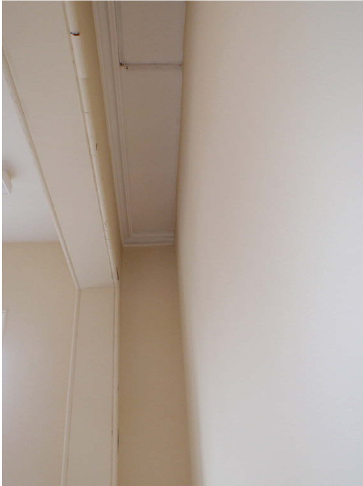
Plate 15 Interview room 2, cut-through wall and ceiling edge moulding crossed by inserted modern partition wall
