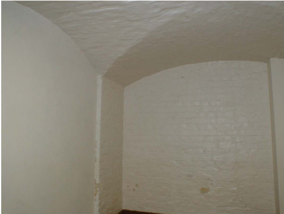
Plate 19 Cells. Note difference of painted brick in alcove to right and smooth rendered finish in alcove to left
