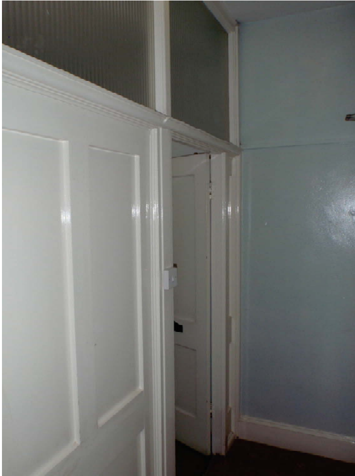
Plate 1 1 st Floor WC, from corridor, panel wall with borrowed light glazing
