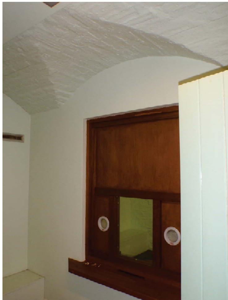
Plate 20 Cells 'interview room'. Note smooth rendered finish of wall around communication panel
