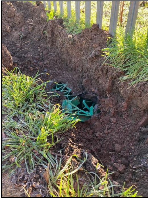
Existing Soakaway alongside Site Access
