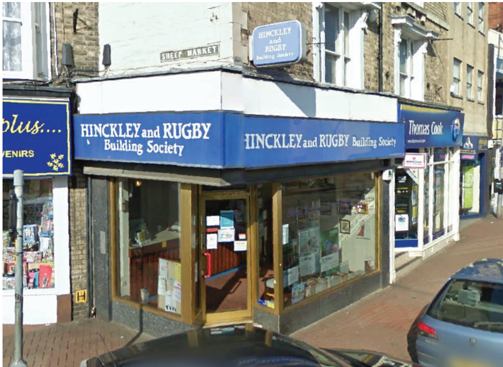
Spalding Branch Before:
