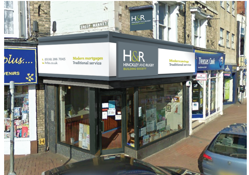
Spalding Branch After:
