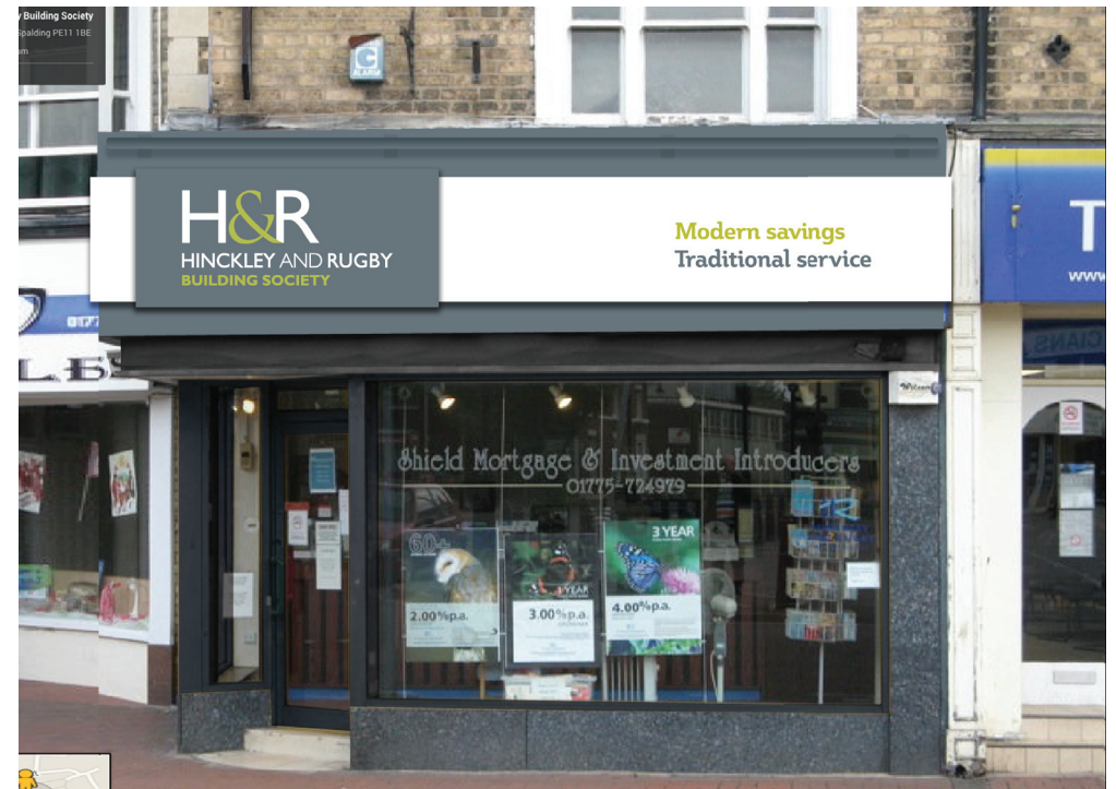
Spalding Branch After:
