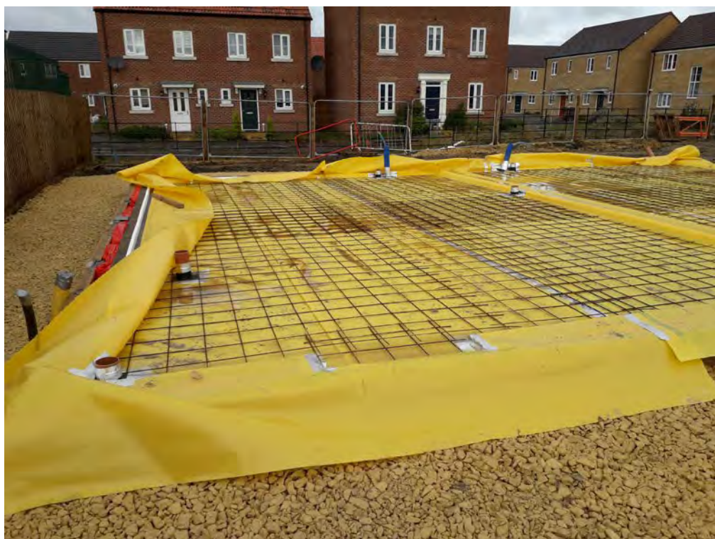
Photo 1 – General view across Plot 910/911.
