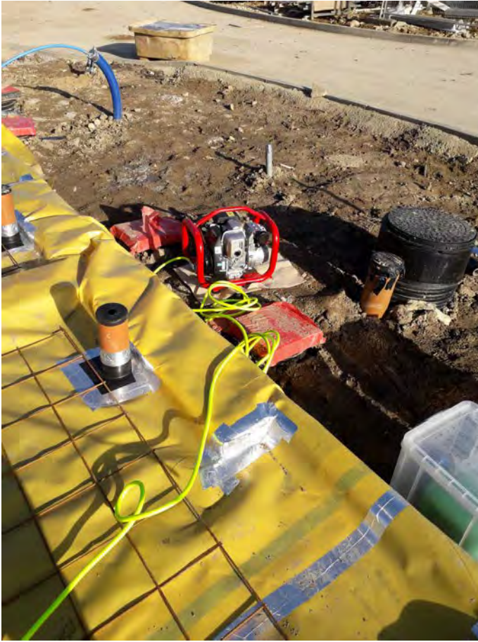
Photo 3 – Detail of tape seals around a corner joint and top hat.
