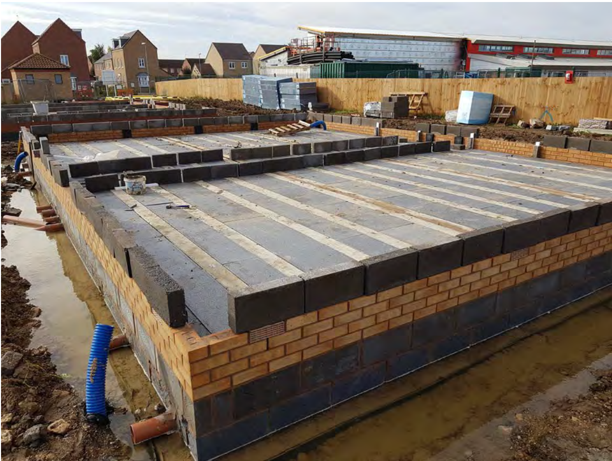
Photo 6 – Plots 908/909 showing air bricks and periscopic vents. Thick layer of final insulation yet to be laid upon which the membrane will be fitted. Not plot 904 in distance with yellow membrane.
