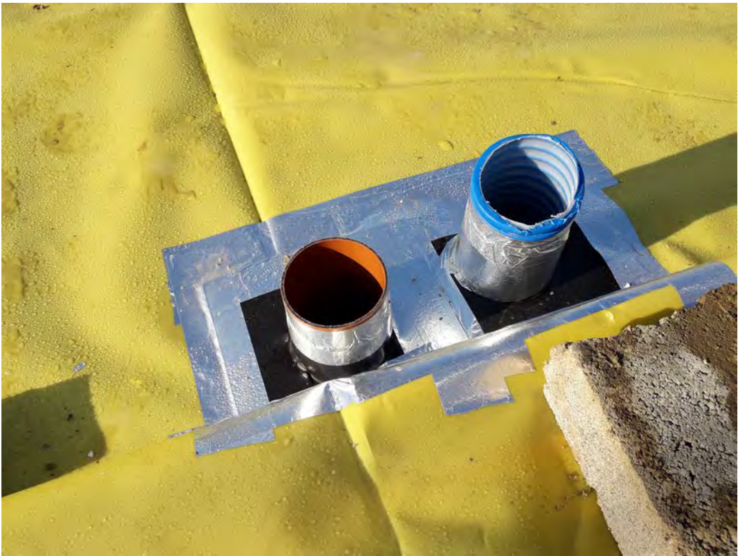
Photo 3 – Minor tear in corner of corner joint due to wind lifting membrane.
