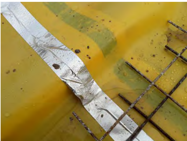
Photo 3 – Break in seal at lap up onto outer brick wall and following repair.
