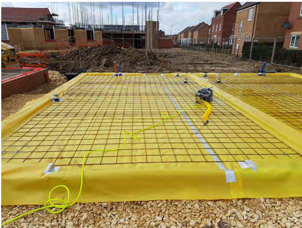
Photo 1 – General view across Plot 924/925.
