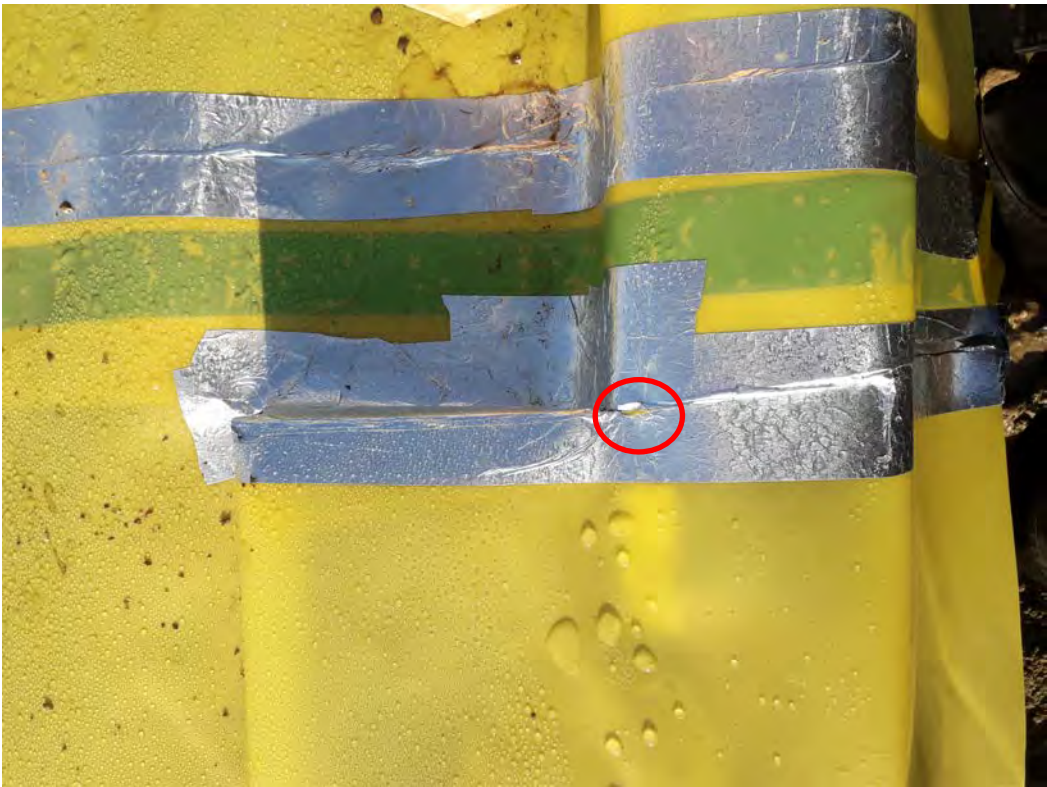
Photo 3 – Minor tear in corner of corner joint due to wind lifting membrane.
