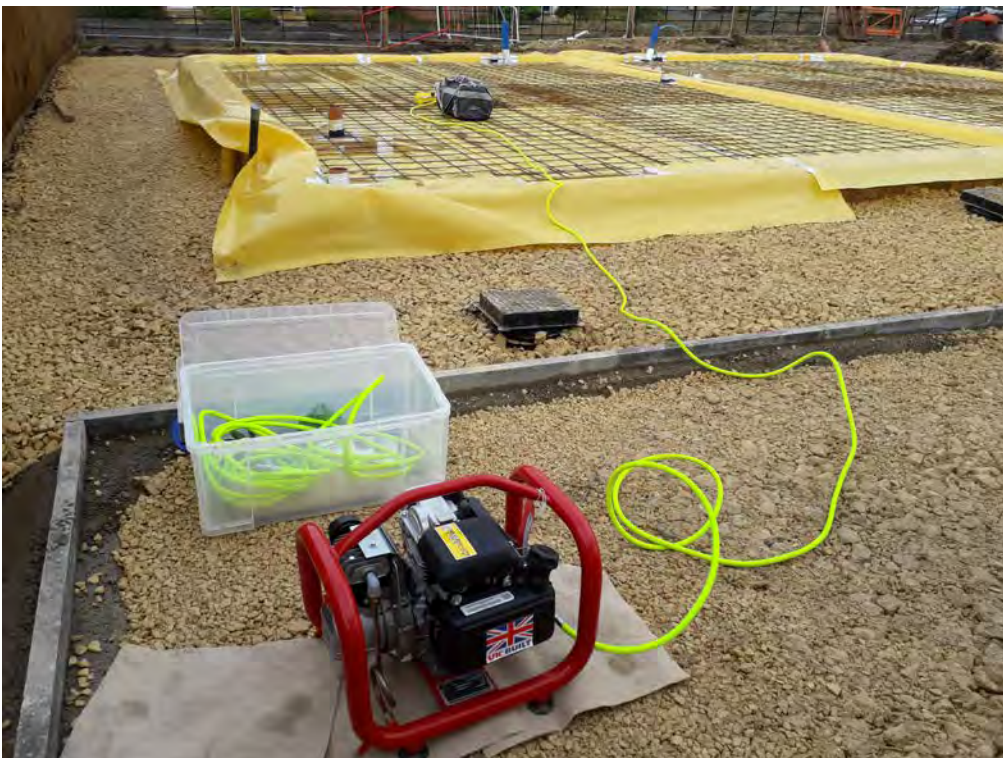
Photo 5 – Use of air lance testing to check the integrity of the membrane.
