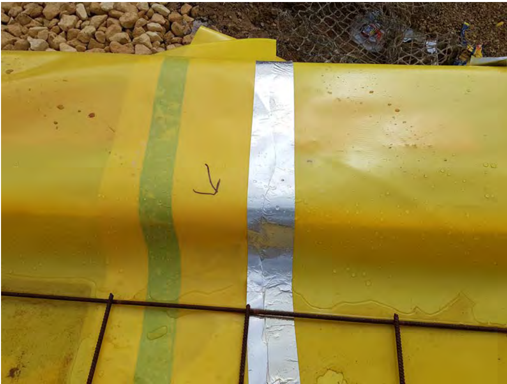
Photo 3 – View of membrane to stairwell of Plot 923. Note air lance used during verification.
