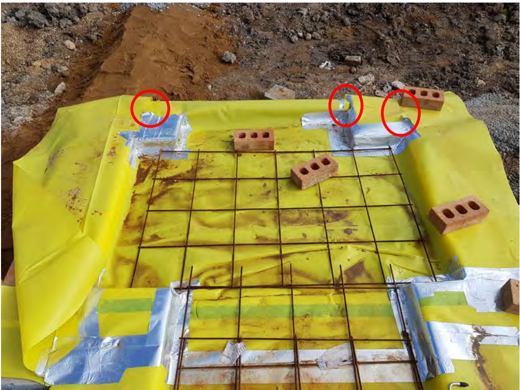
Photo 7 – Corner detailing for Plot 926, note three identified defects within silver tape corner seal.
