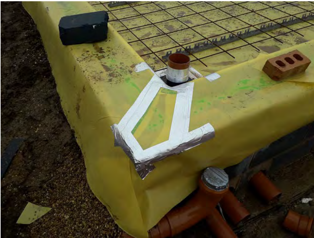
Photo 6 – Corner of Plot 901 following repair.
