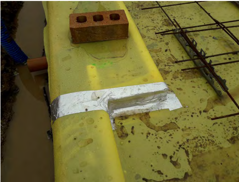
Photo 3 – Detail of sealing around top hats which were all to a good standard. Note loose jubilee clip not tightened by the fitters due to concern clips might compromise the taped seal.
