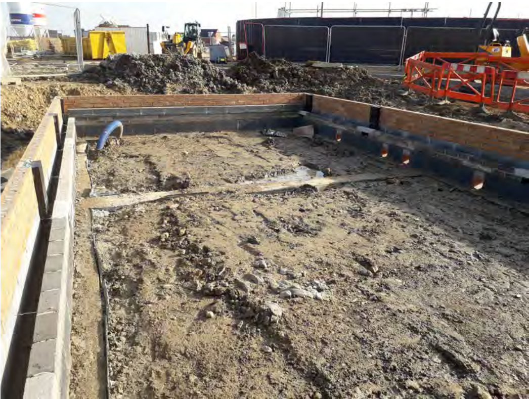
Photo 6 – Close up of interior of Plot 920 showing void and periscopic ducts.
