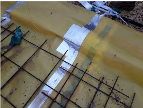
Photo 3 – Break in seal at lap up onto outer brick wall and following repair.
