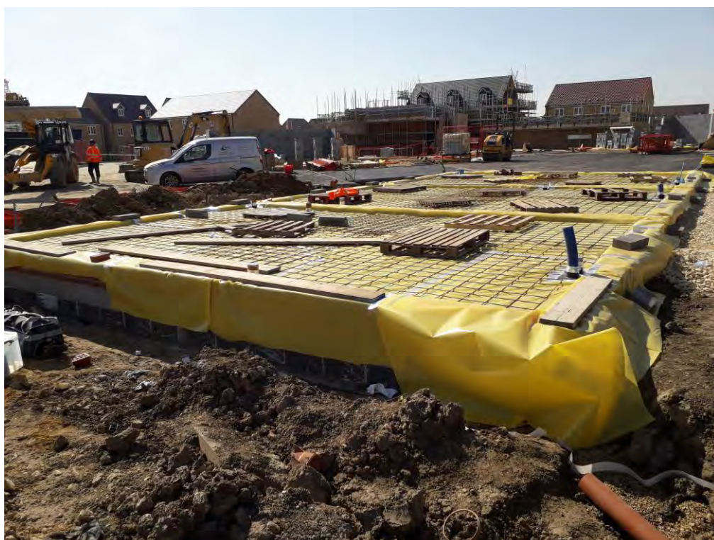
Photo 1 - General view across Plot 927/928/929.
