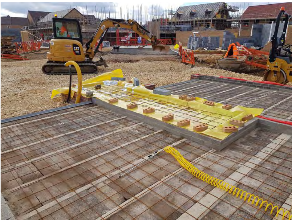
Photo 3 – View of membrane to stairwell of Plot 923. Note air lance used during verification.
