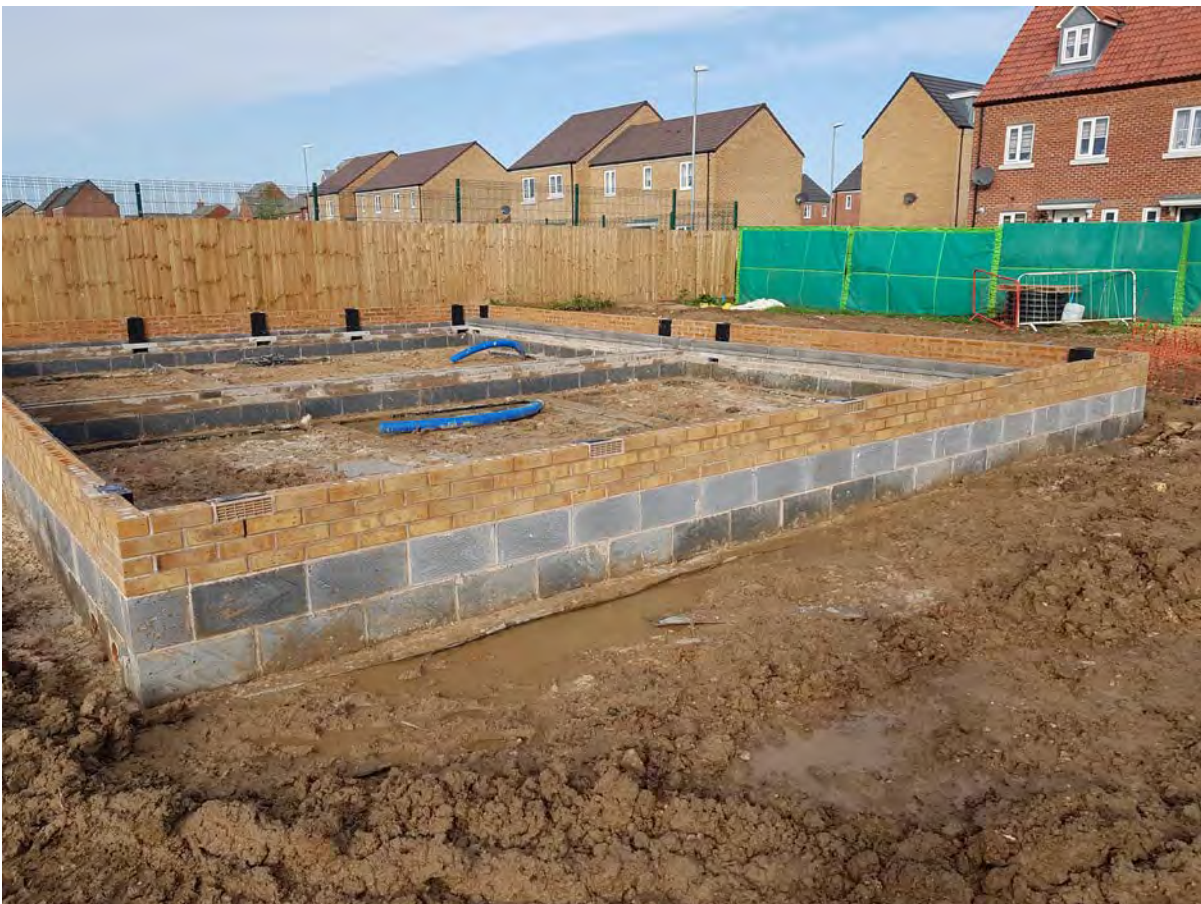
Photo 5 – Plot 910/911 before placement of beams showing ready void and periscopic vents.
