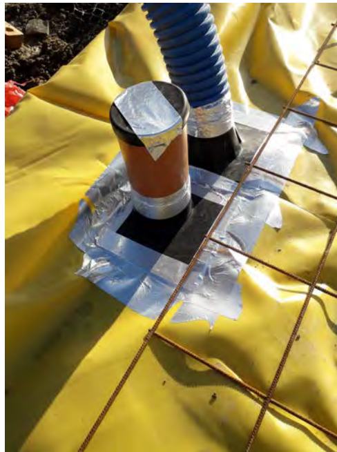
Photo 5 – Patch repairs on the membrane placed prior to the inspection visit.
