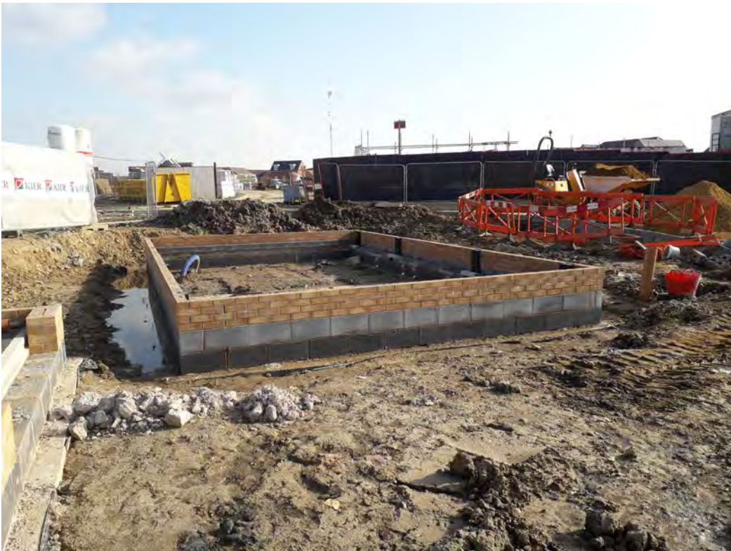
Photo 5 – Plot 920 showing void, air bricks and periscopic ducts.
