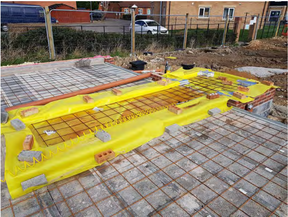
Photo 7 – Corner detailing for Plot 926, note three identified defects within silver tape corner seal.
