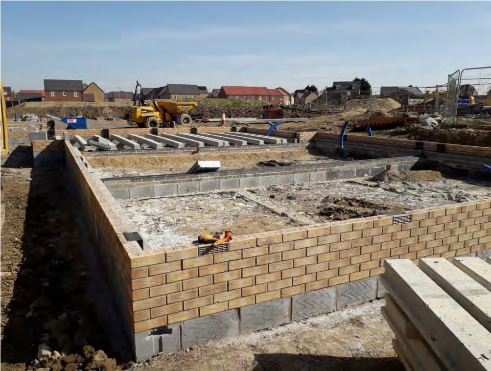
Photo 3 - General view of Plot 933/934 showing air brick along external walls.
