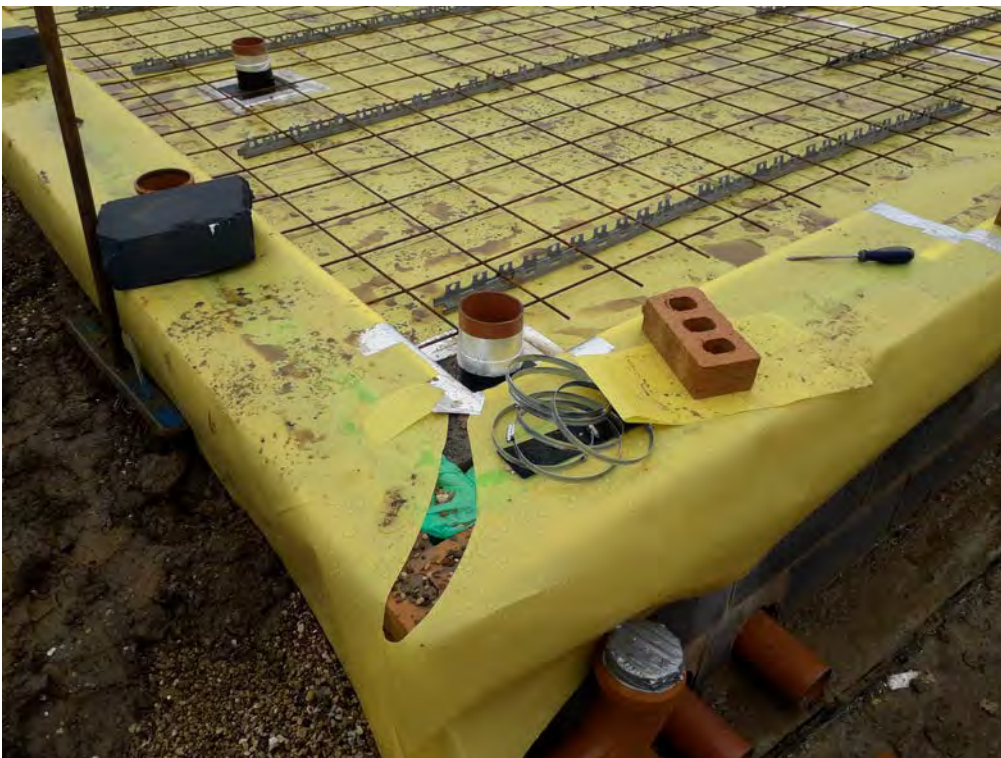
Photo 5 – Tear in the corner of Plot 901. Note material nearby to enable a repair.
