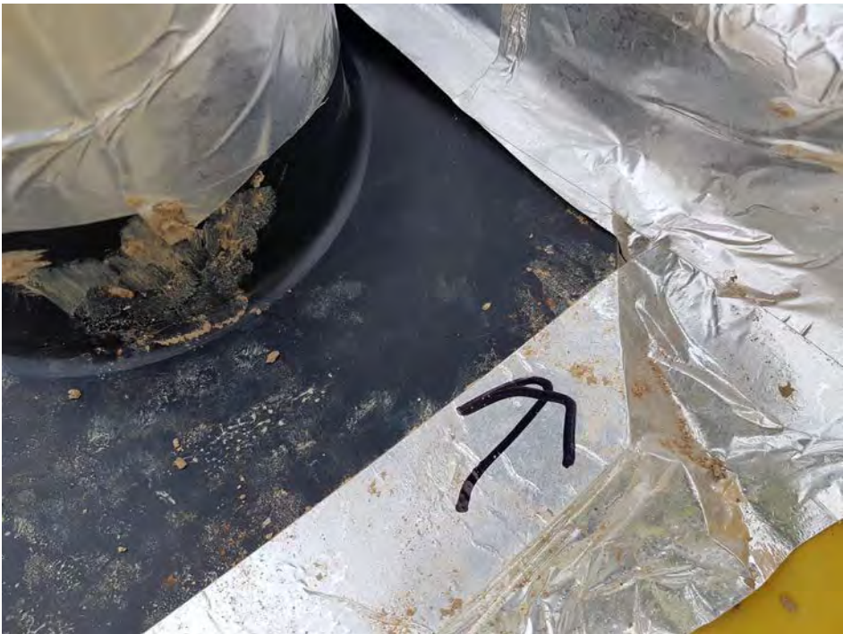
Photo 4 - Defect around top hat before repair.
