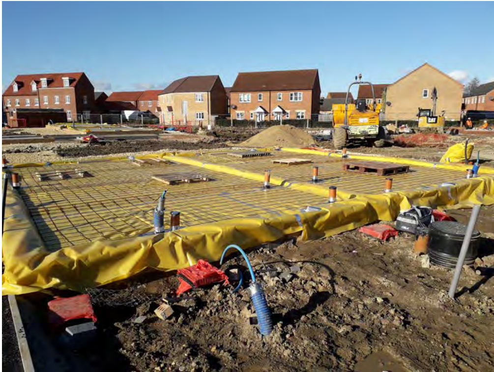
Photo 1 – General view across Plot 921/922.
