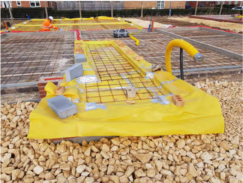
Photo 5 – Minor defect on tape seal for Plot 923.
