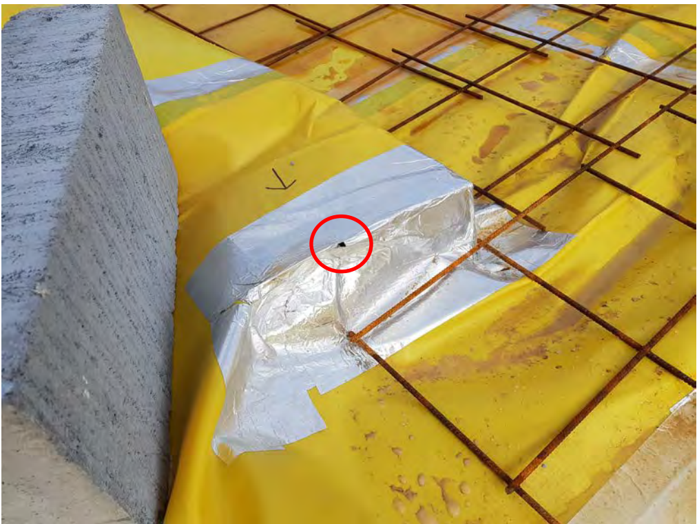
Photo 5 – Minor defect on tape seal for Plot 923.
