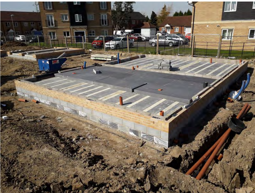
Photo 3 - General view of Plot 933/934 showing air brick along external walls.
