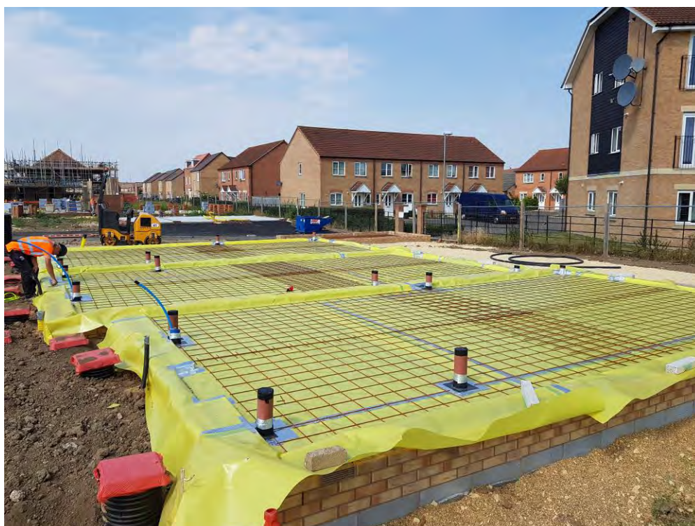
Photo 1 - General view across Plot 930/931/932.
