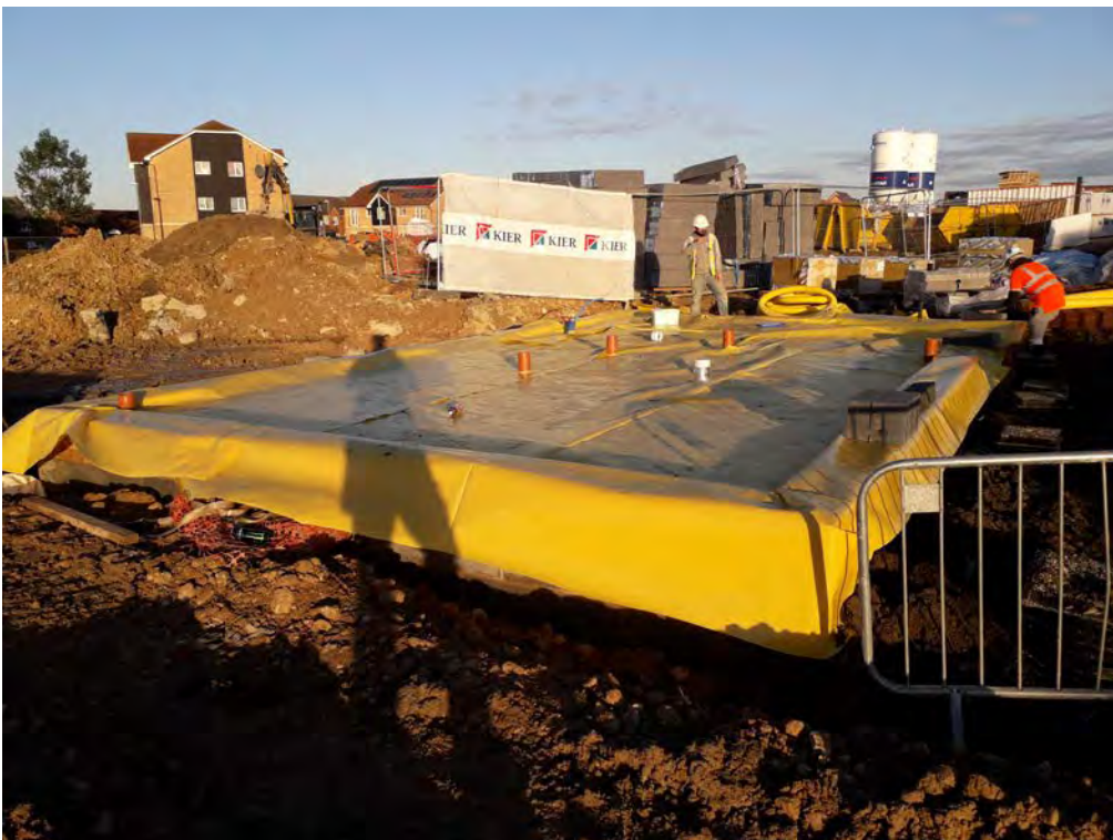
Photo 7 – Plot 920 showing ongoing installation of membrane.
