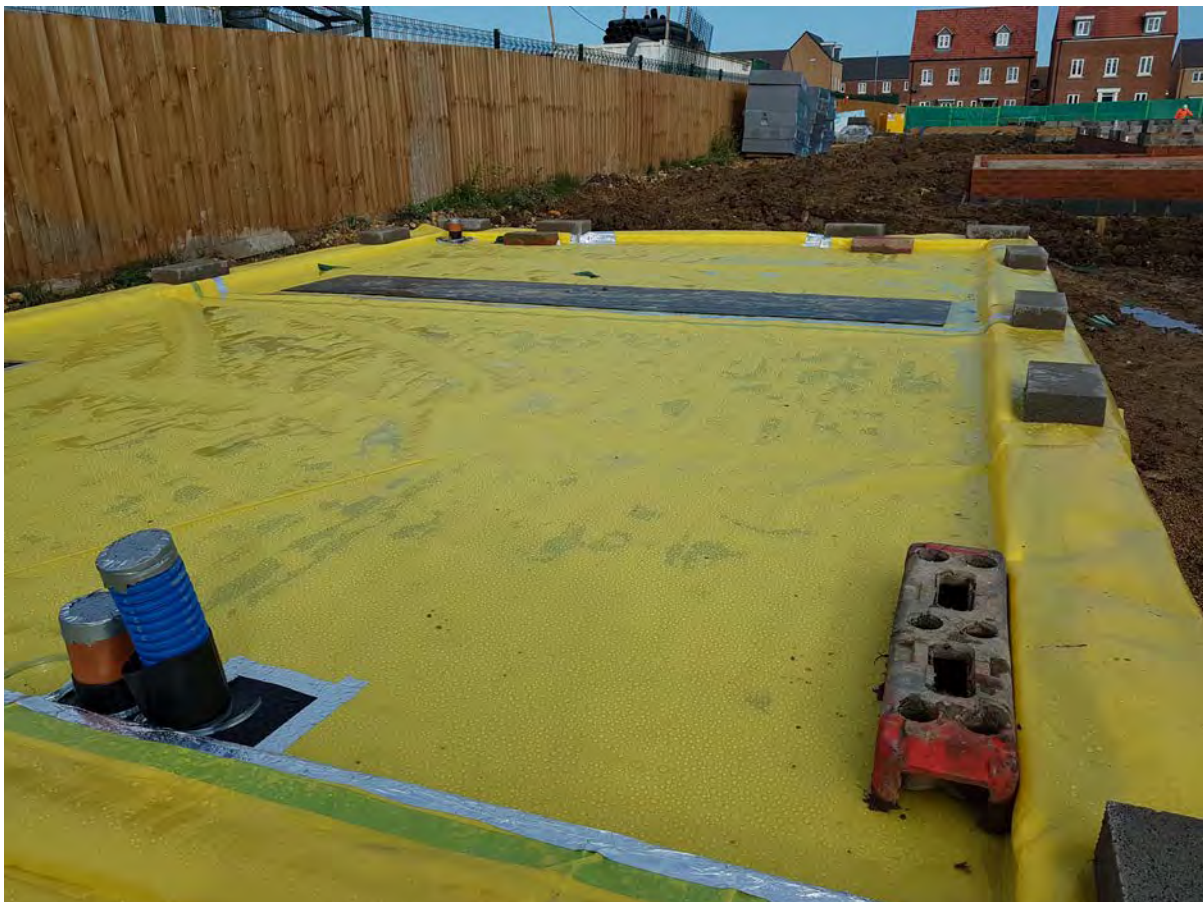
Photo 3 – Plot 904, the first plot to have the membrane fitted. Note black crawl board used when fitting central joint left in place for the purpose of the verification inspection.
