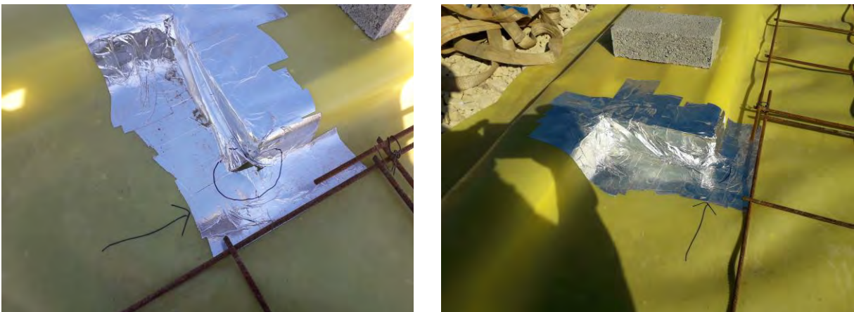
Photo 5 - Tear in silver tape within a corner joint before and after repair.
