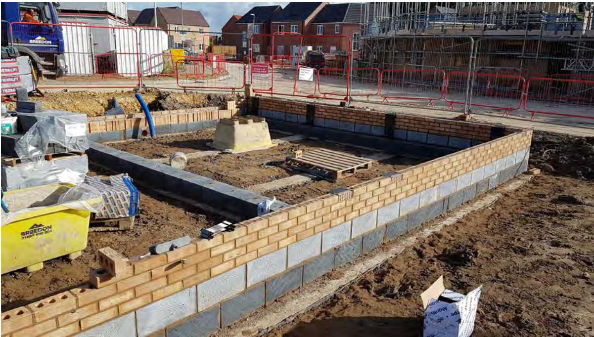
Photo 8 – Plots 901 to 903 under construction showing air bricks and void.
