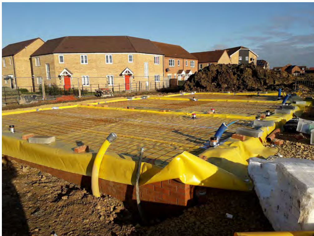
Photo 1 – General view across Plot 912/913/914.
