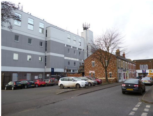
Fig. 07 – The Telephone Exchange to the West.
