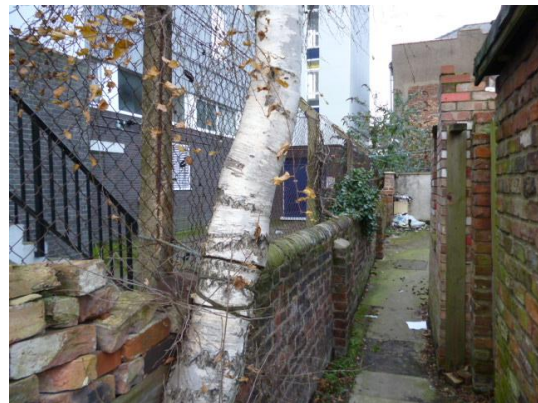
Fig. 6 – Garden wall on the west boundary.
