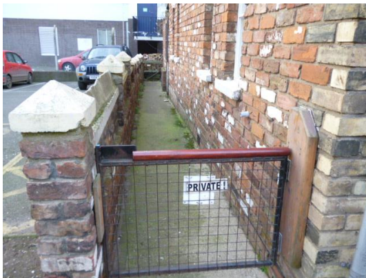
Fig. 05 – Boundary wall to the south.
