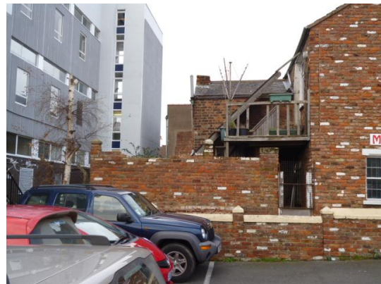
Fig. 02 – Partly developed rear yard area.
