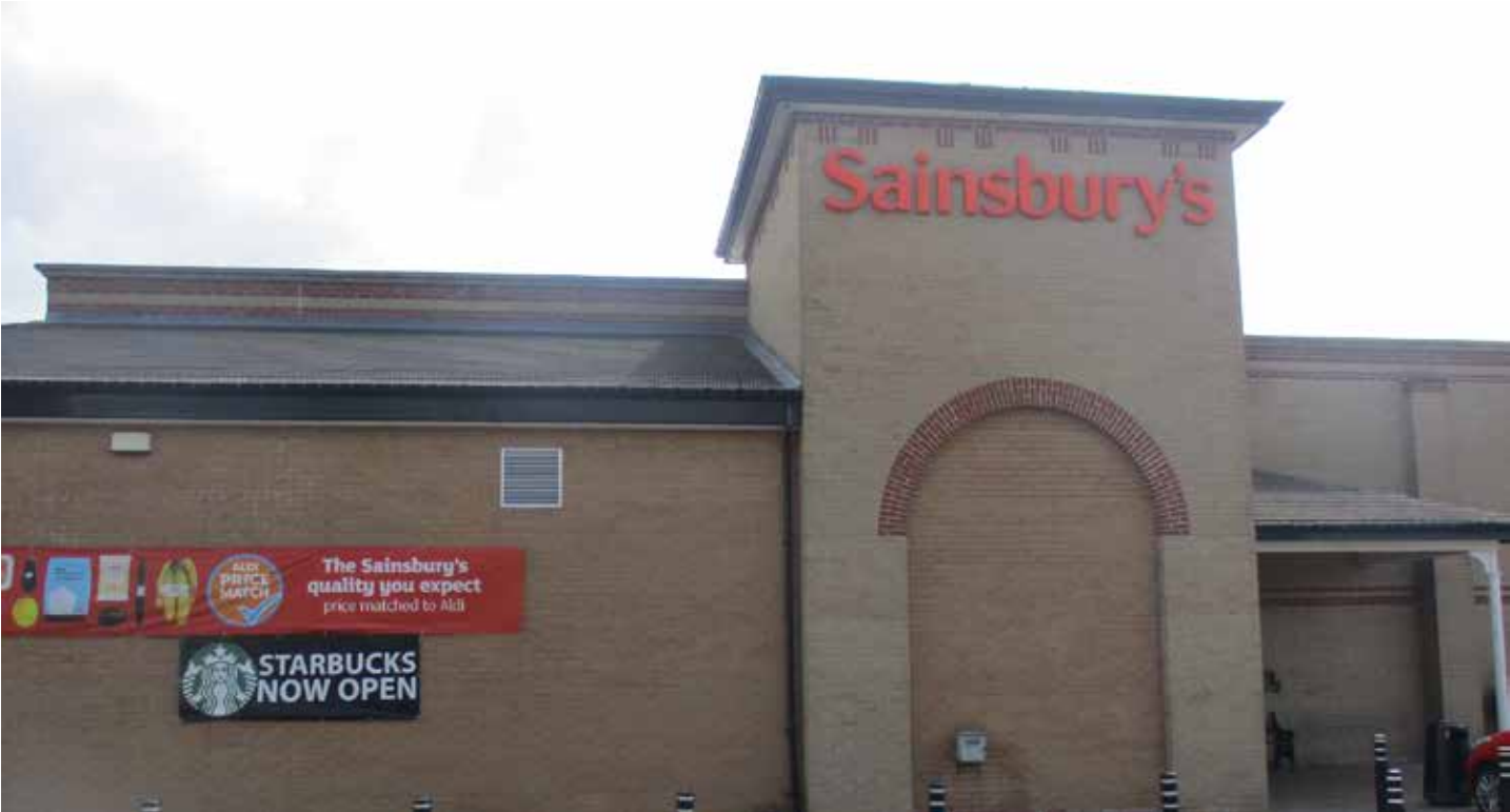
Elevation C - Existing View
