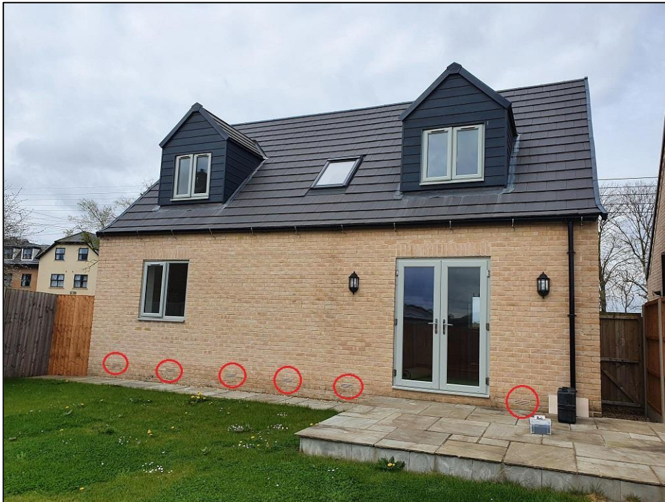
Figure 1 Sub-floor void air bricks on eastern side of property.
