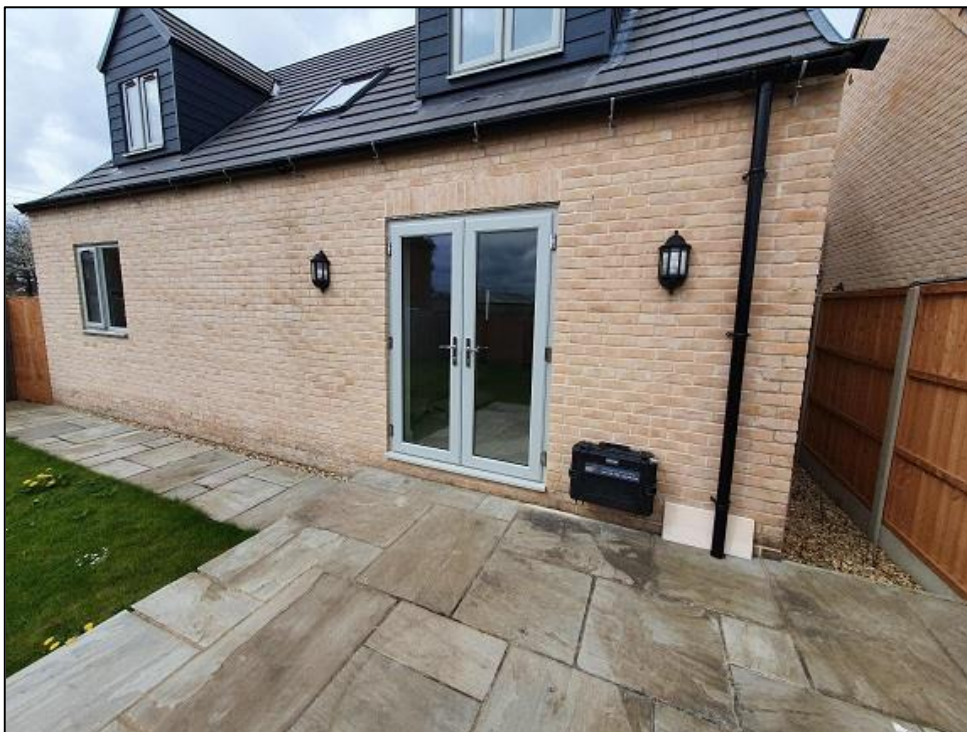
Figure 2 GGS site photograph of the Gas Sentinel® instrumentation installed and secured on site.
