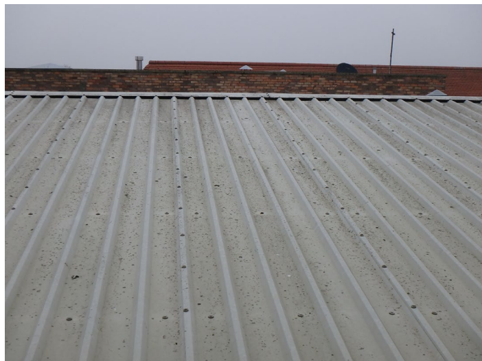
View over adjacent roof, looking north
