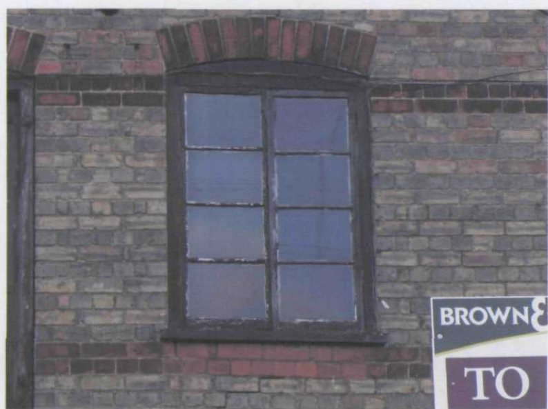
First Floor Window - Swan Street Elevation
