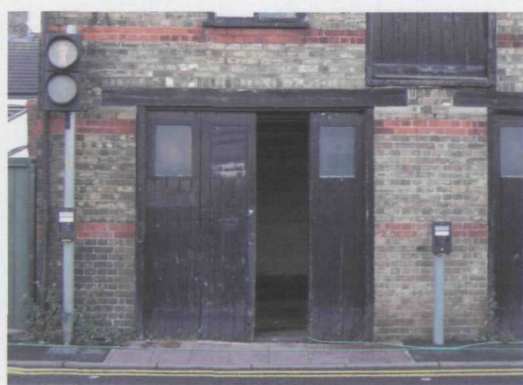
Existing Entrance Door - Swan Street Elevation
