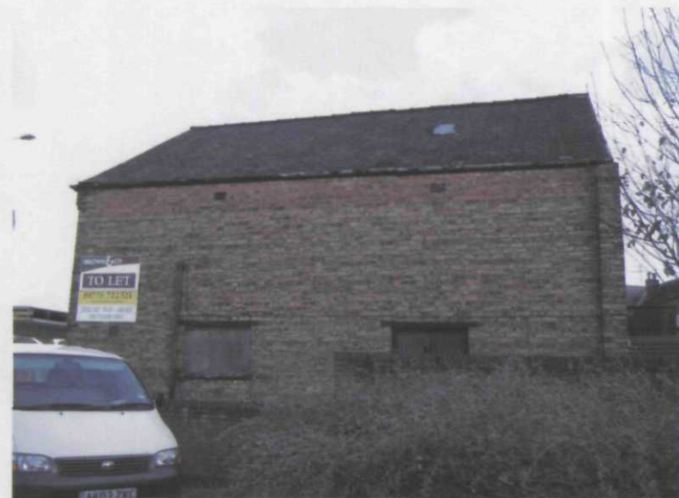
Elevation to adjacent pedestrian area
