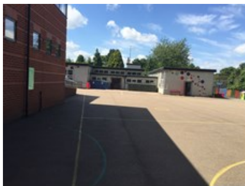
Fig. 02 – Annex block in the west corner of the site.
