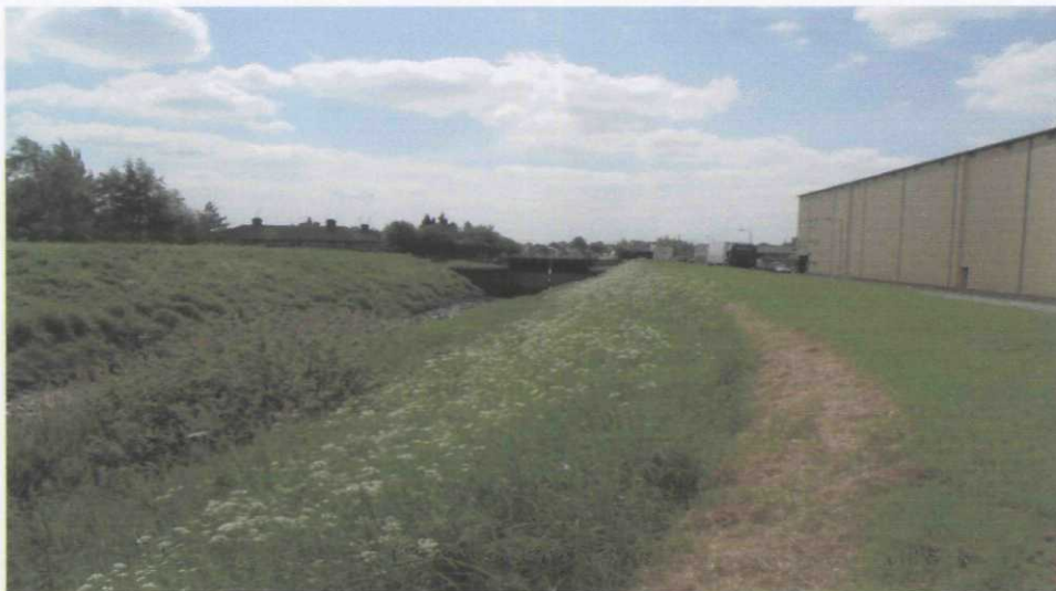
MARSH ROAD SLUICE – TIDAL / FLUVIAL RIVER WELLAND
