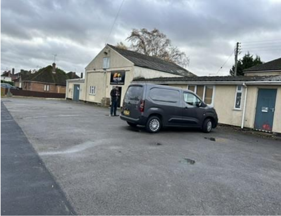
Photograph 3: Further view of the hardstanding and building
