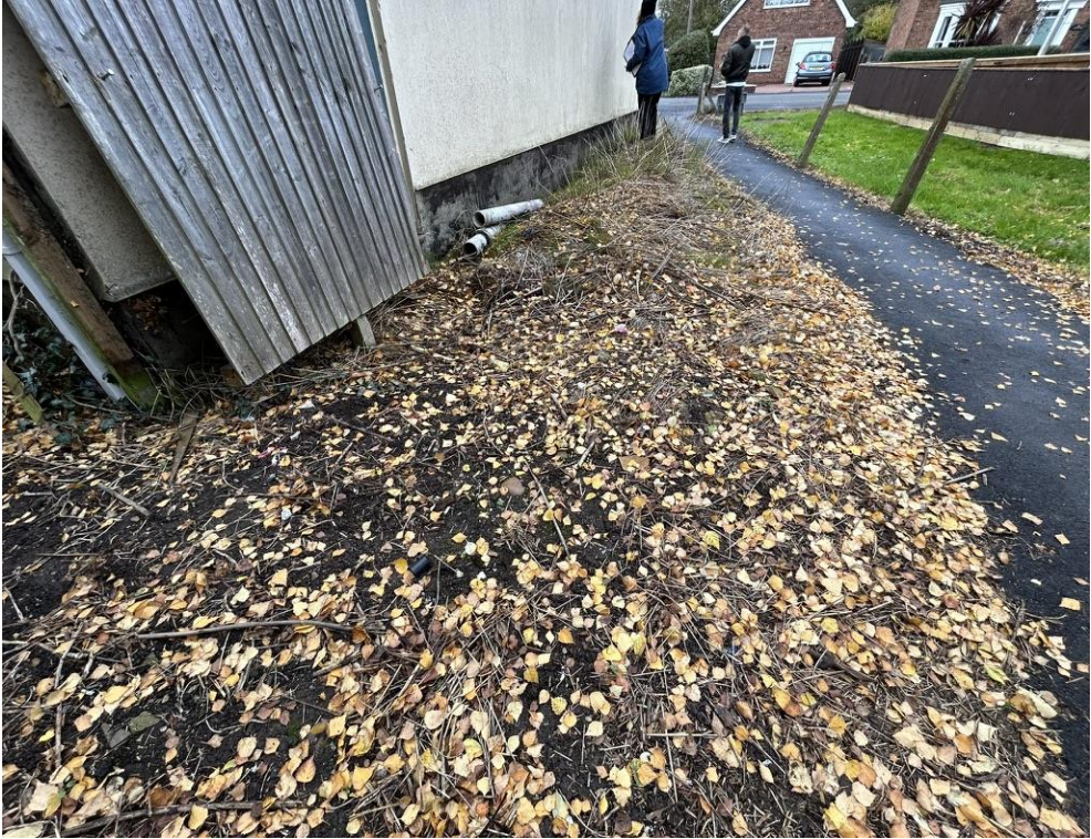
Photograph 4: Unvegetated unsealed surface to the east of the building
