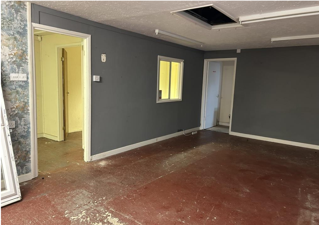
Photograph 9: Ground floor room within the building
