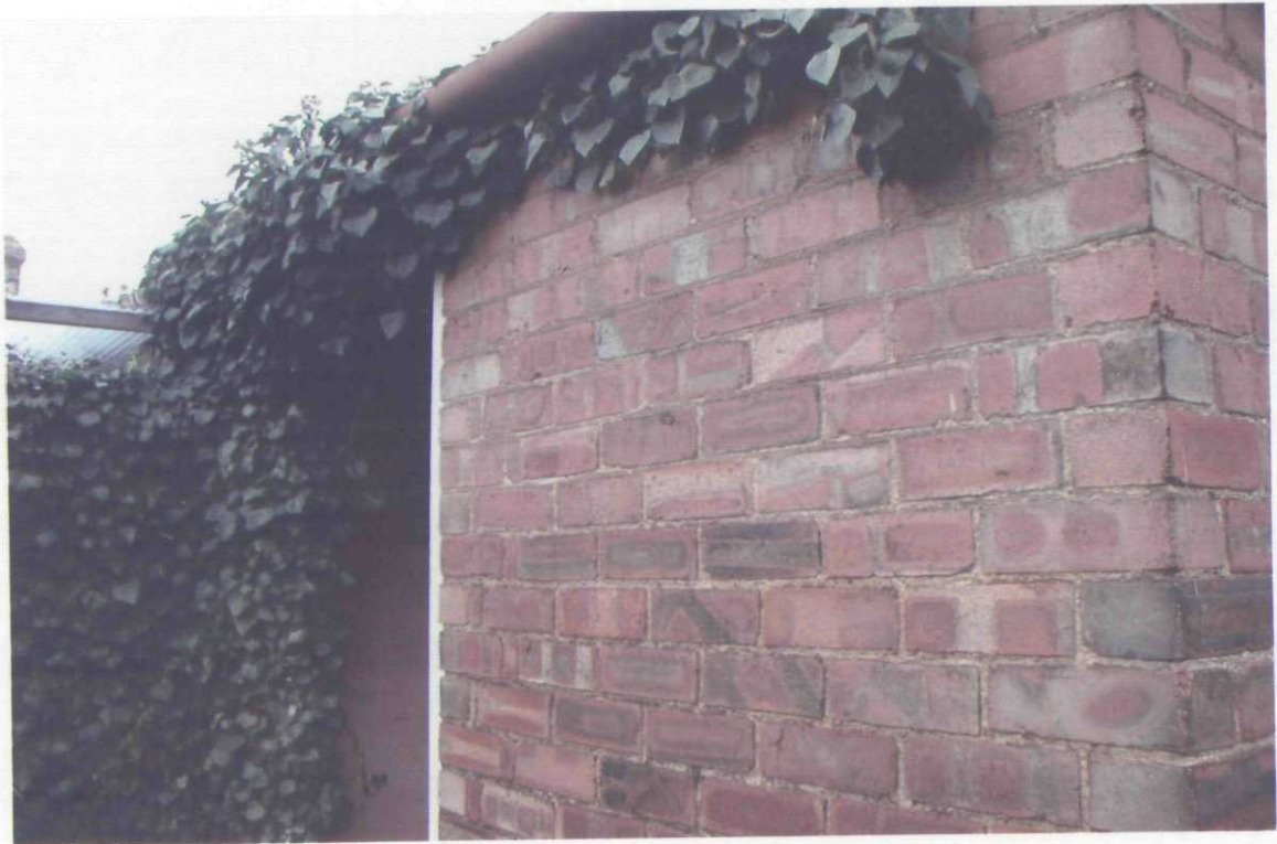
Rear of existing outbuilding & pt. boundary of no 84.
