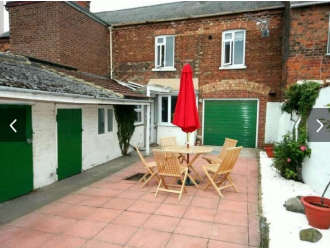
Image 1. The rear of the property in 2012 before some of the single storey outbuildings were removed. Only the far portion of this remains (adjoining the main part of the property). The footprint of the proposed extension will be very similar.
