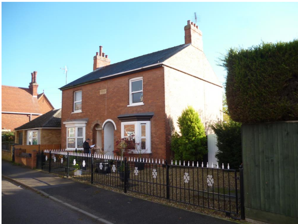
View looking east towards existing building frontage, from South Parade.
