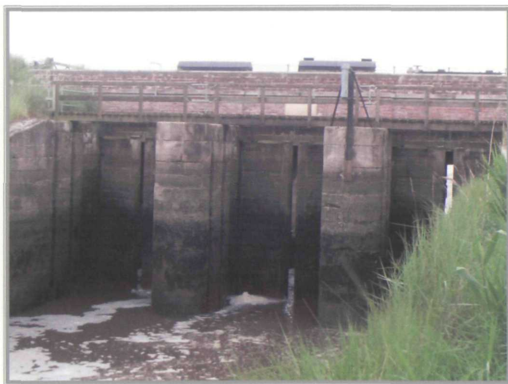
Vernatts Drain Outfall Sluice
