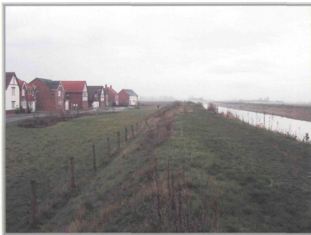
Vernatts Drain Right-hand Embankment adjacent to Sorrel Drive off Wygate Park
