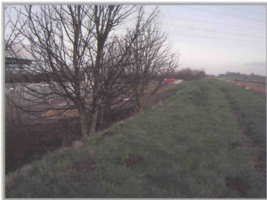
River Welland – Tidal Embankment
