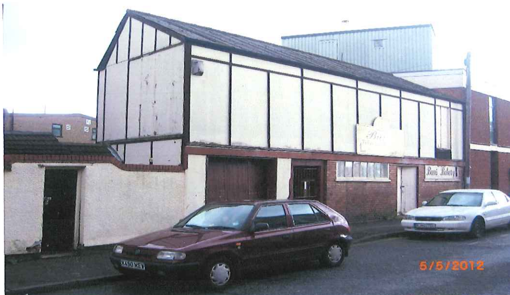
Buildings which stood on the site prior to demolition
